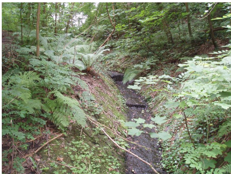
Photographs showing the outflow form the pond to the Cryddan Brook, concreted with laid stone sides
