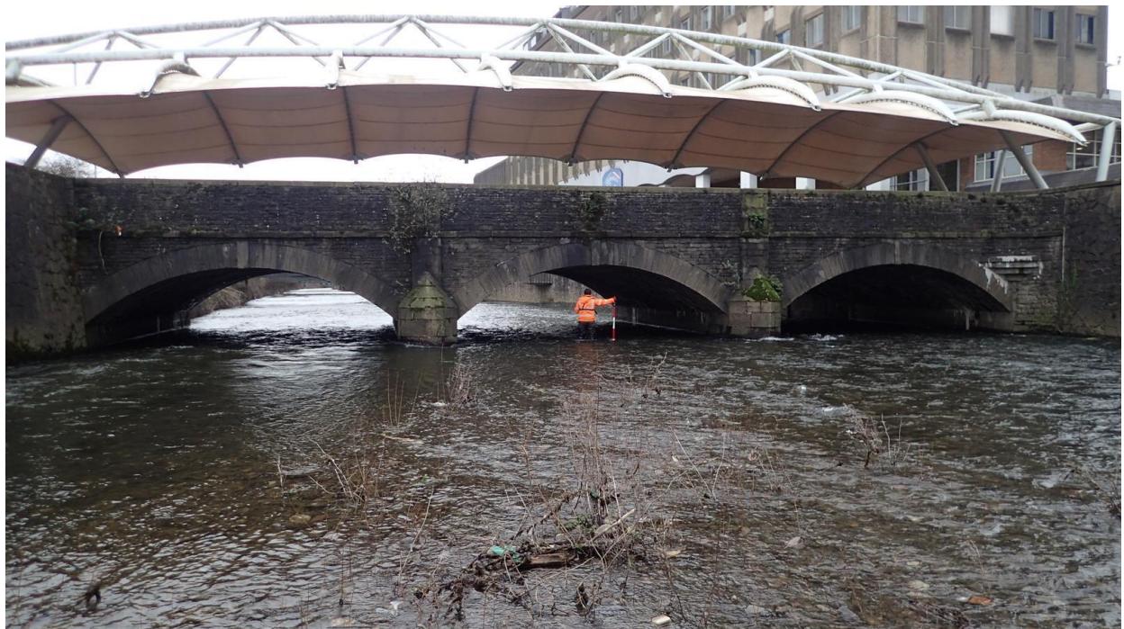
Figure 2-2: Station Road arch bridge
