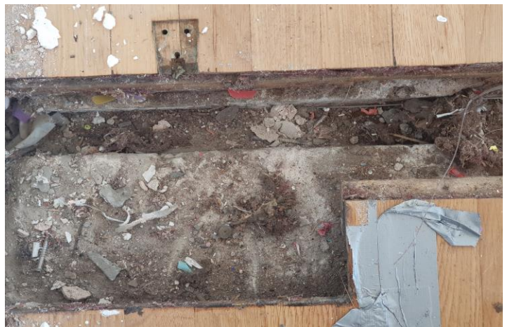
Figure 6, Channel Location in Concrete, beneath timber floor
