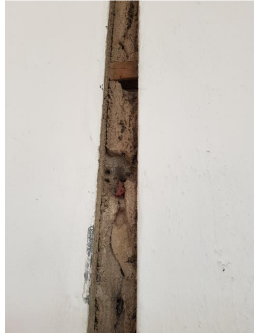
Figure 5, Steel Glazing Channel Removed
