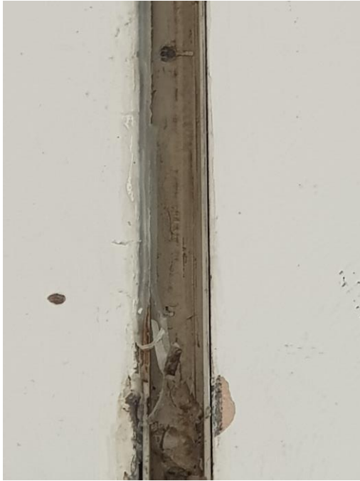
Figure 4, Steel Glazing Channel in Wall
