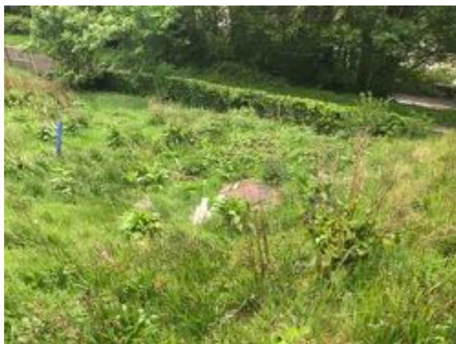
Man hole cover to north of site
