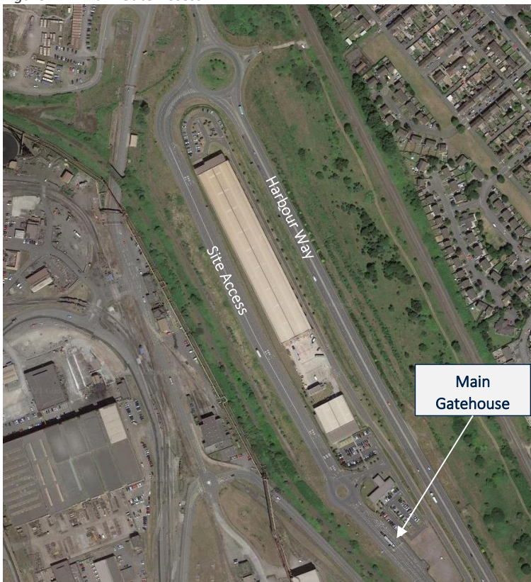
Figure 2-1: Main Gate Access
