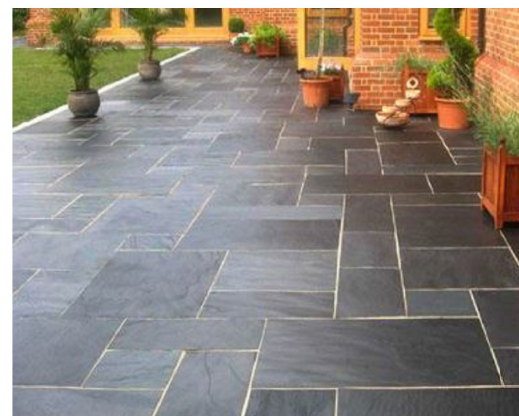
Paving to Driveway & External Paths
