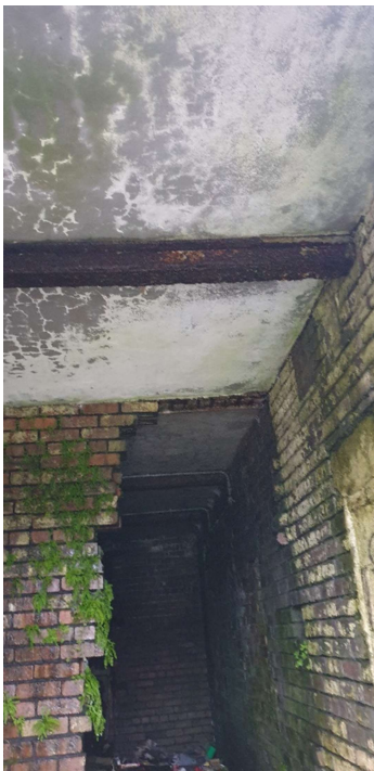
Internal view of the black building.
