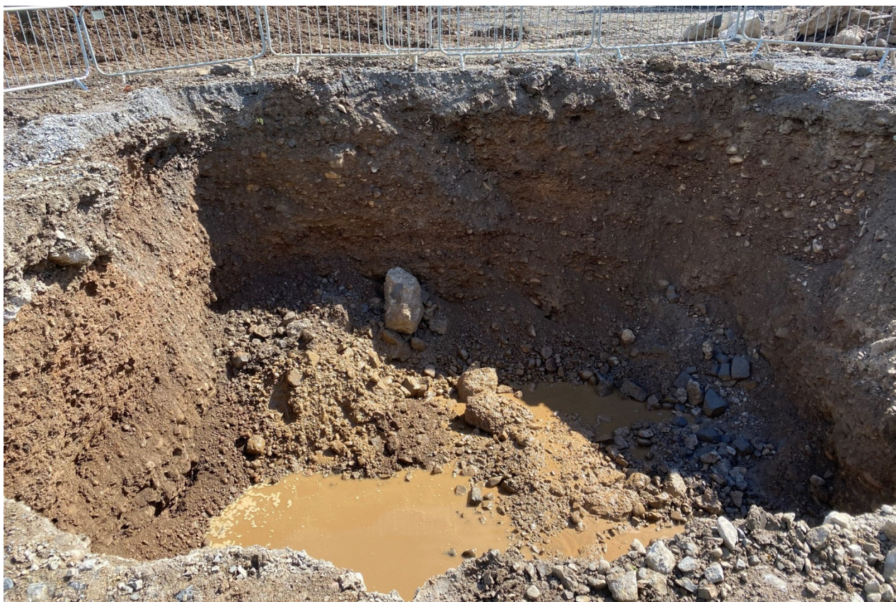
Photograph 6 – Excavation following removal of cradle
