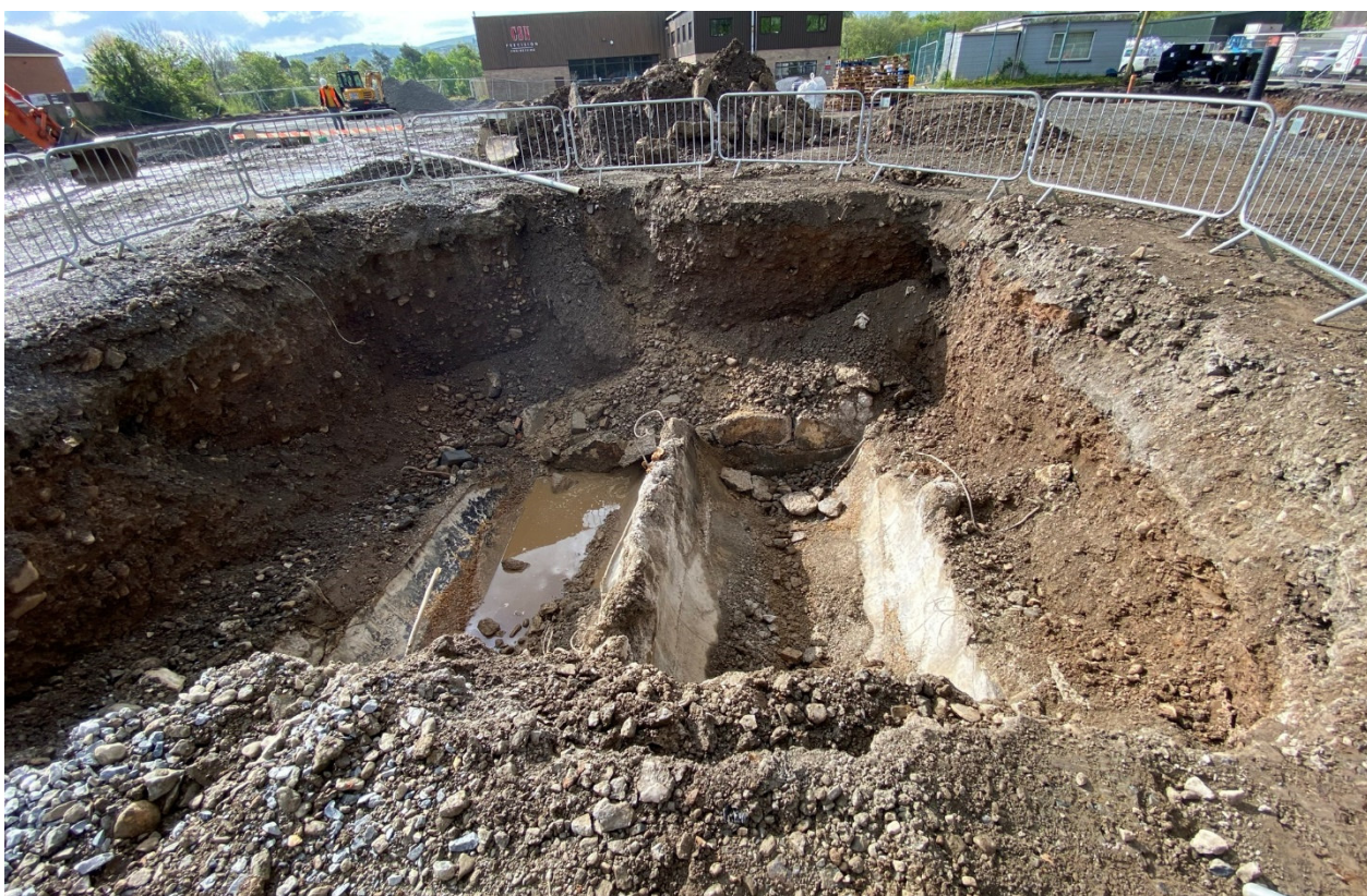
Photograph 4 – Excavation prior to cradle removal
