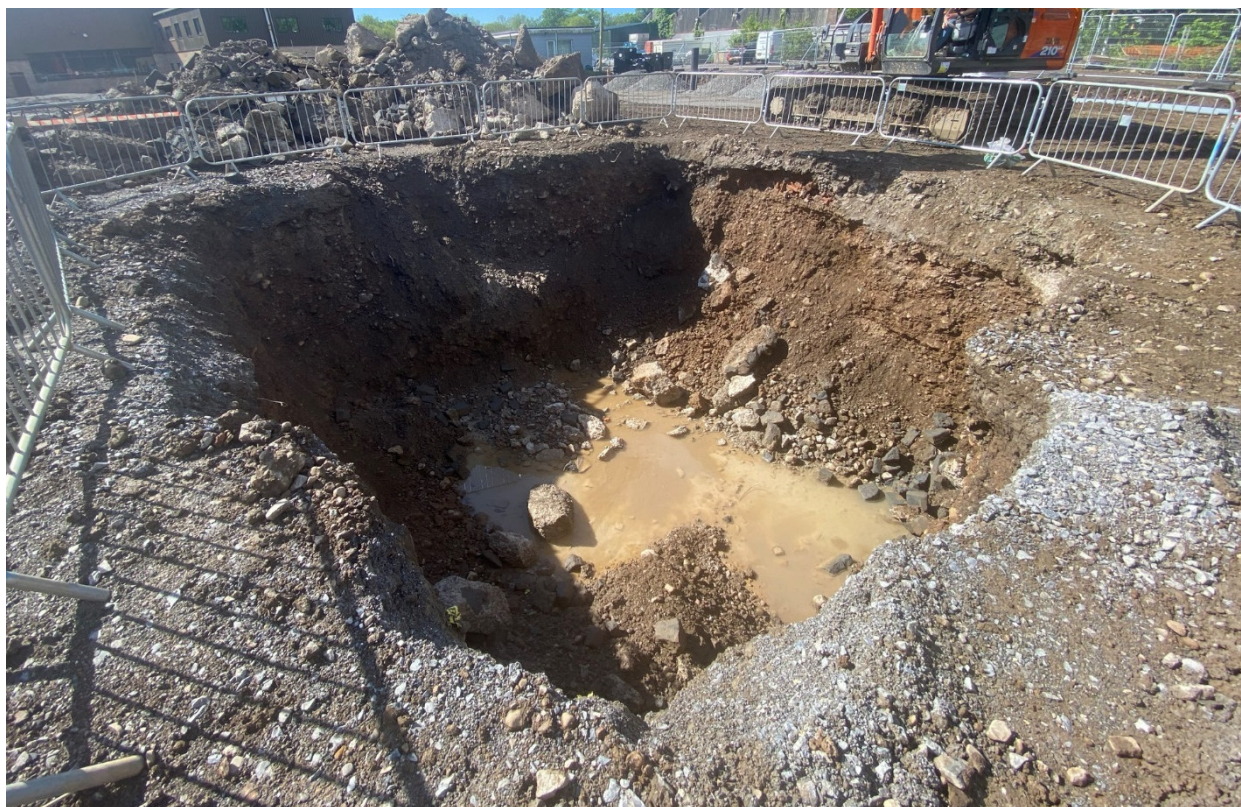
Photograph 5 – Excavation following removal of cradle
