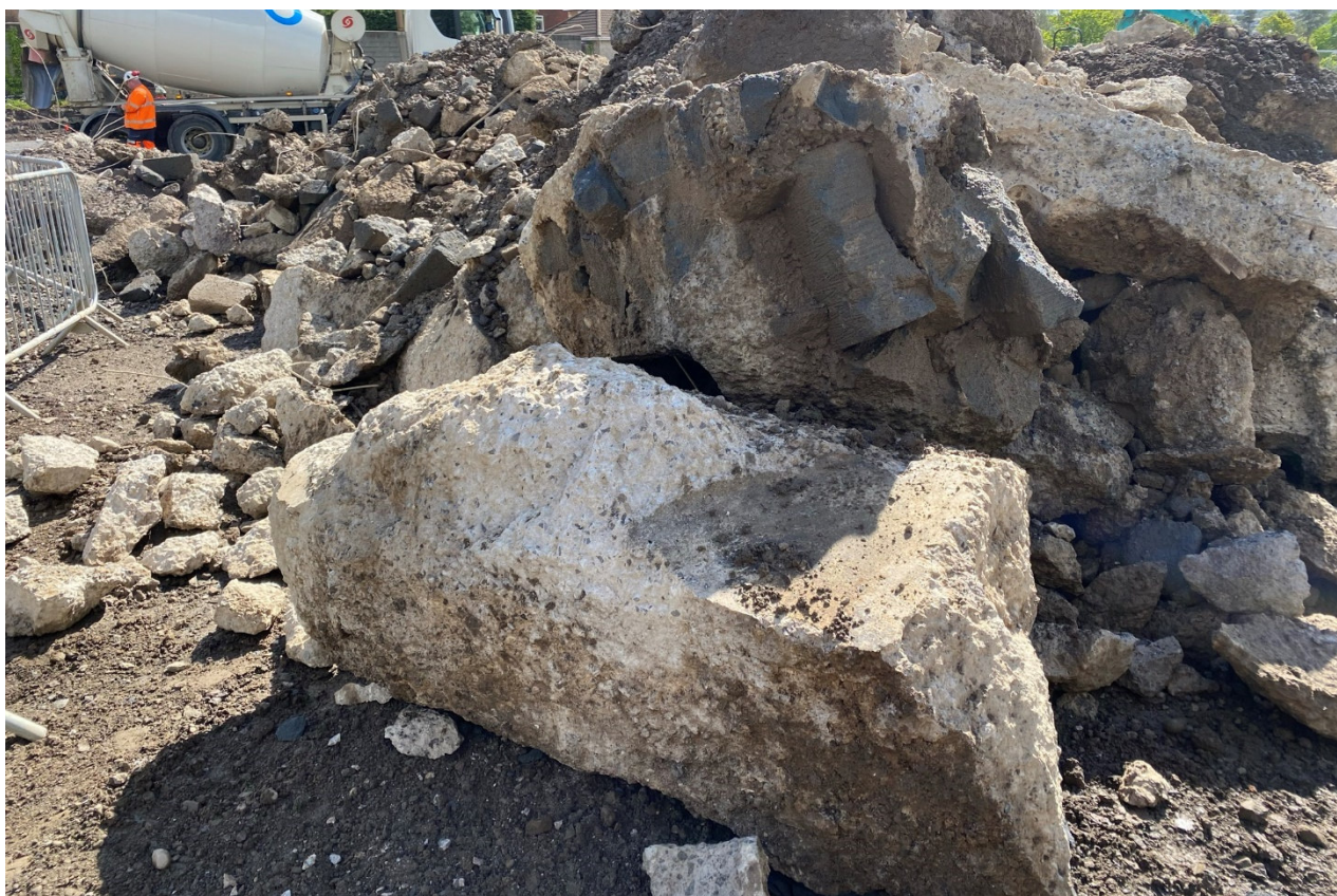
Photograph 8 – Material excavated for disposal.
