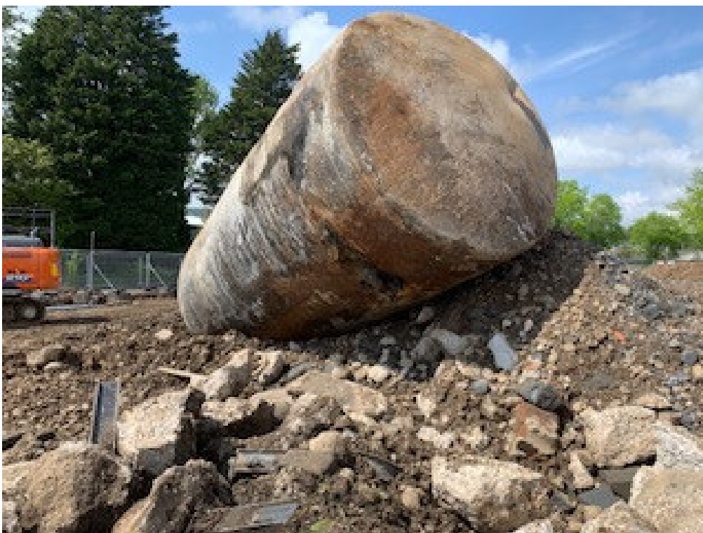
Photograph 2 – Removed tank
