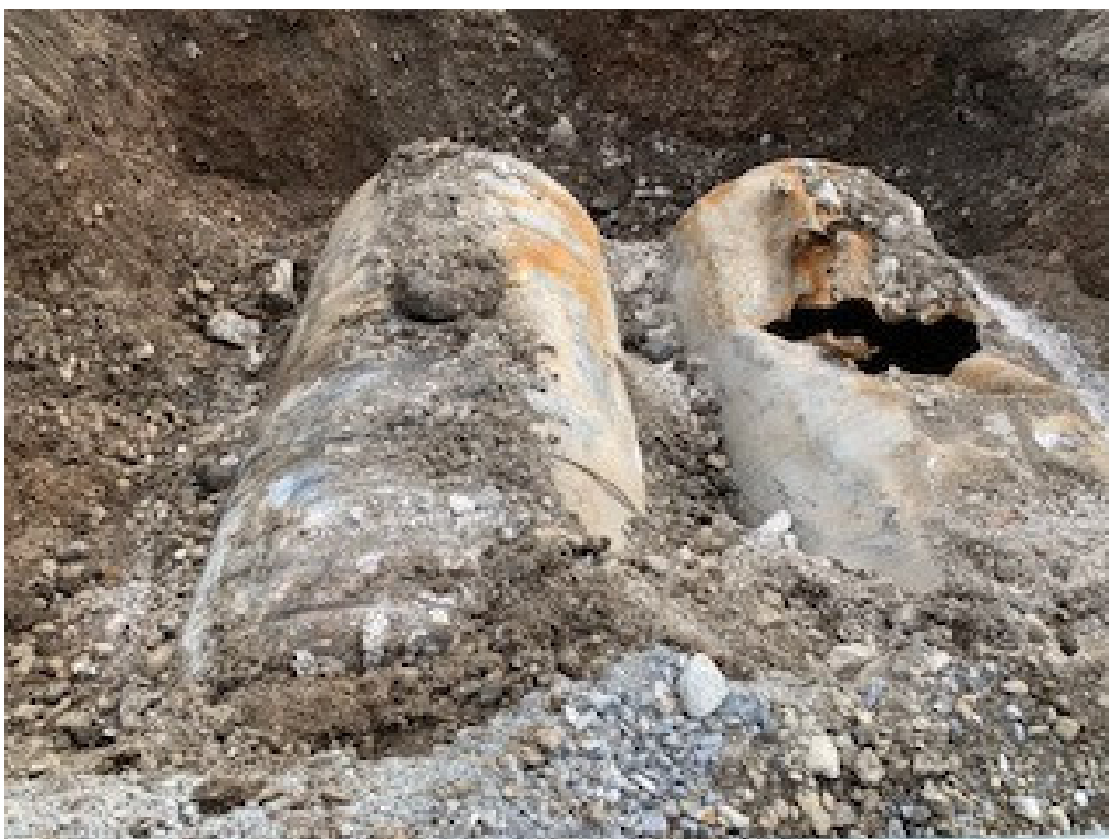
Photograph 1 – USTs in situ prior to exhumation
