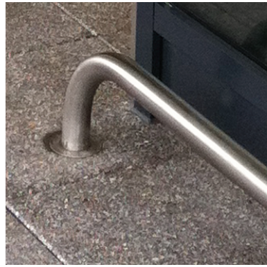
1 Trolley Rails and Protection Rails, brushed stainless steel sections (grade 316) - Satin polished finish
