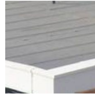
5 Roof - Kingspan 'Topdeck' KS1000/71/TD/ECOSAFE with composite membrane.
