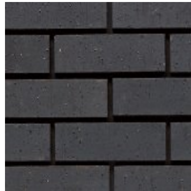
7 Blockleys brick Ltd. 'smooth black' with tarmac y14 (black) coloured mortar brickwork to plinth
