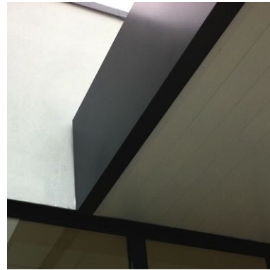
2 Canopy cladding - polyester powder coated aluminium, colour - dark grey ral 7016 (anthracite)
