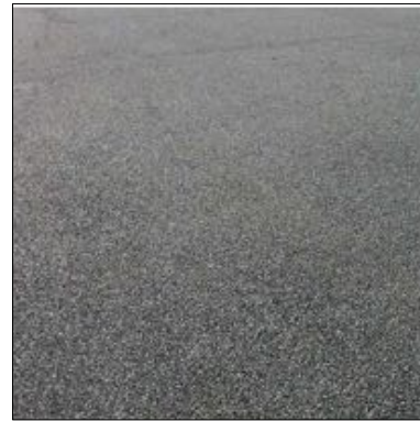
5 Tarmac beneath Aldi canopy
