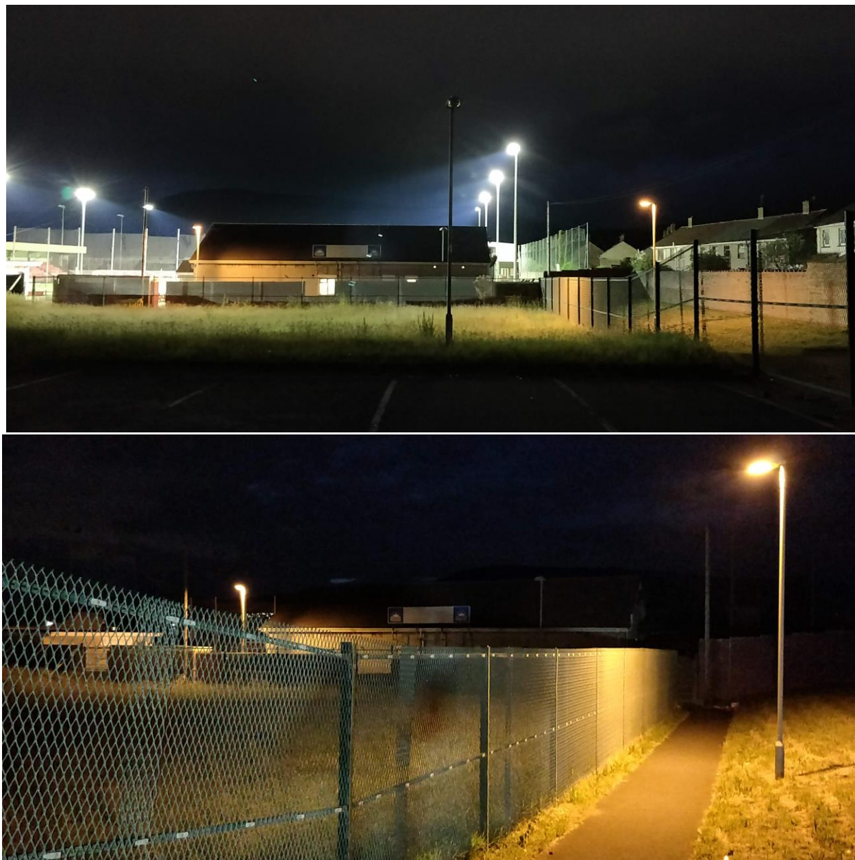
Figure 3-13 – Security Street Lighting at Proposed Residential Development Site with LED Floodlighting On and Off
