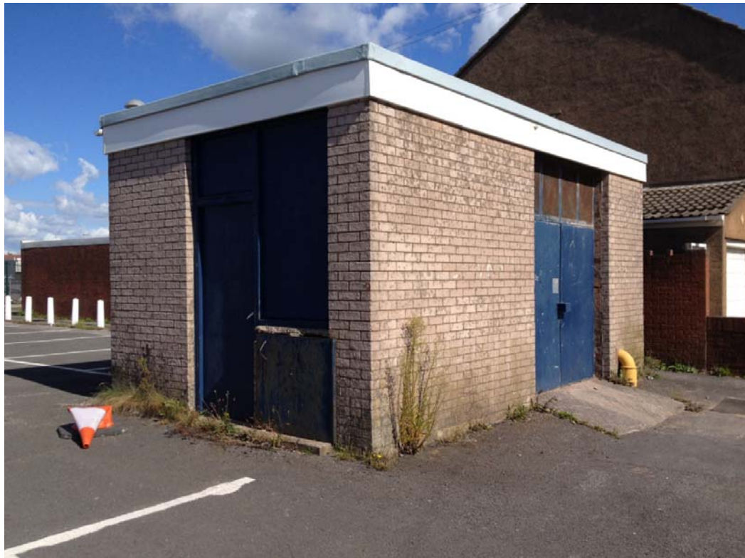
Plate 8 – Gas governor in eastern corner of lido site
