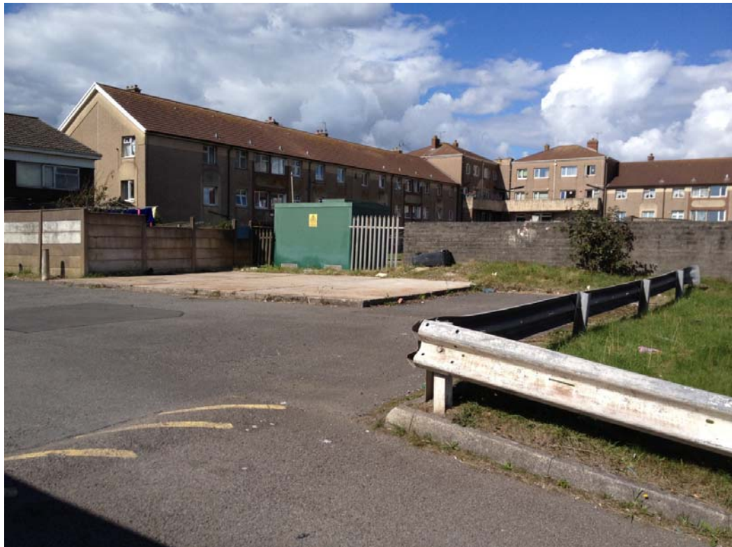
Plate 33 – Substation 30m to the north
