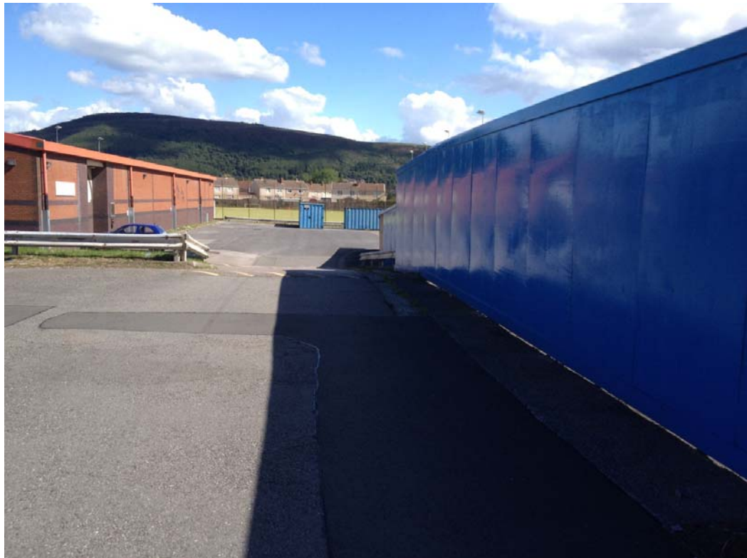
Plate 31 – Indoor bowls centre off northern corner
