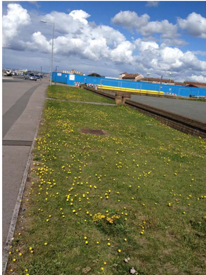
Plate 26 – Drainage along southwest
