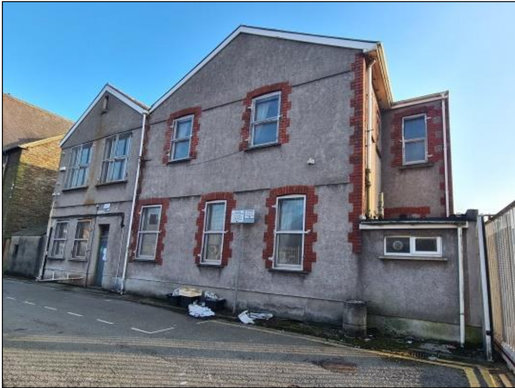
Photo 4. The Rear Elevation of the Proposed Development Site
