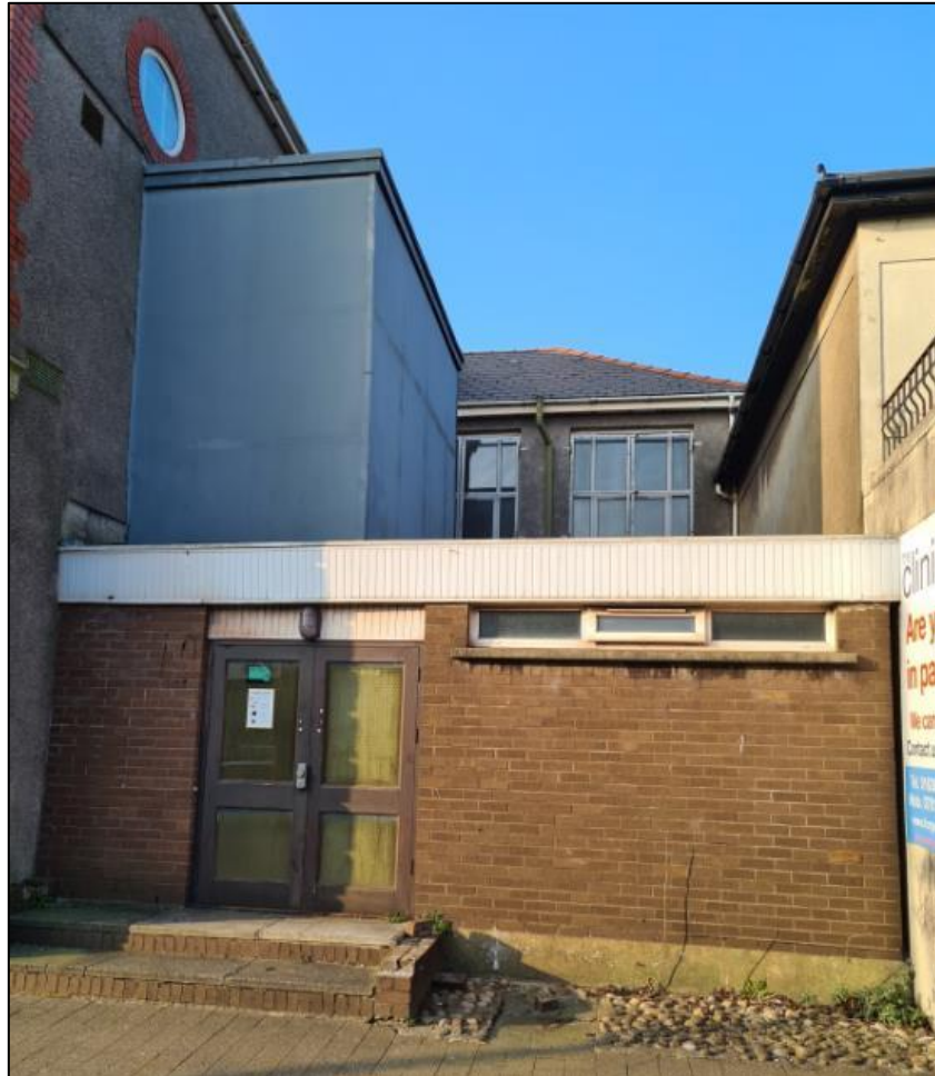
Photo 3. The Late 20 th Century Extensions to the East Elevation
