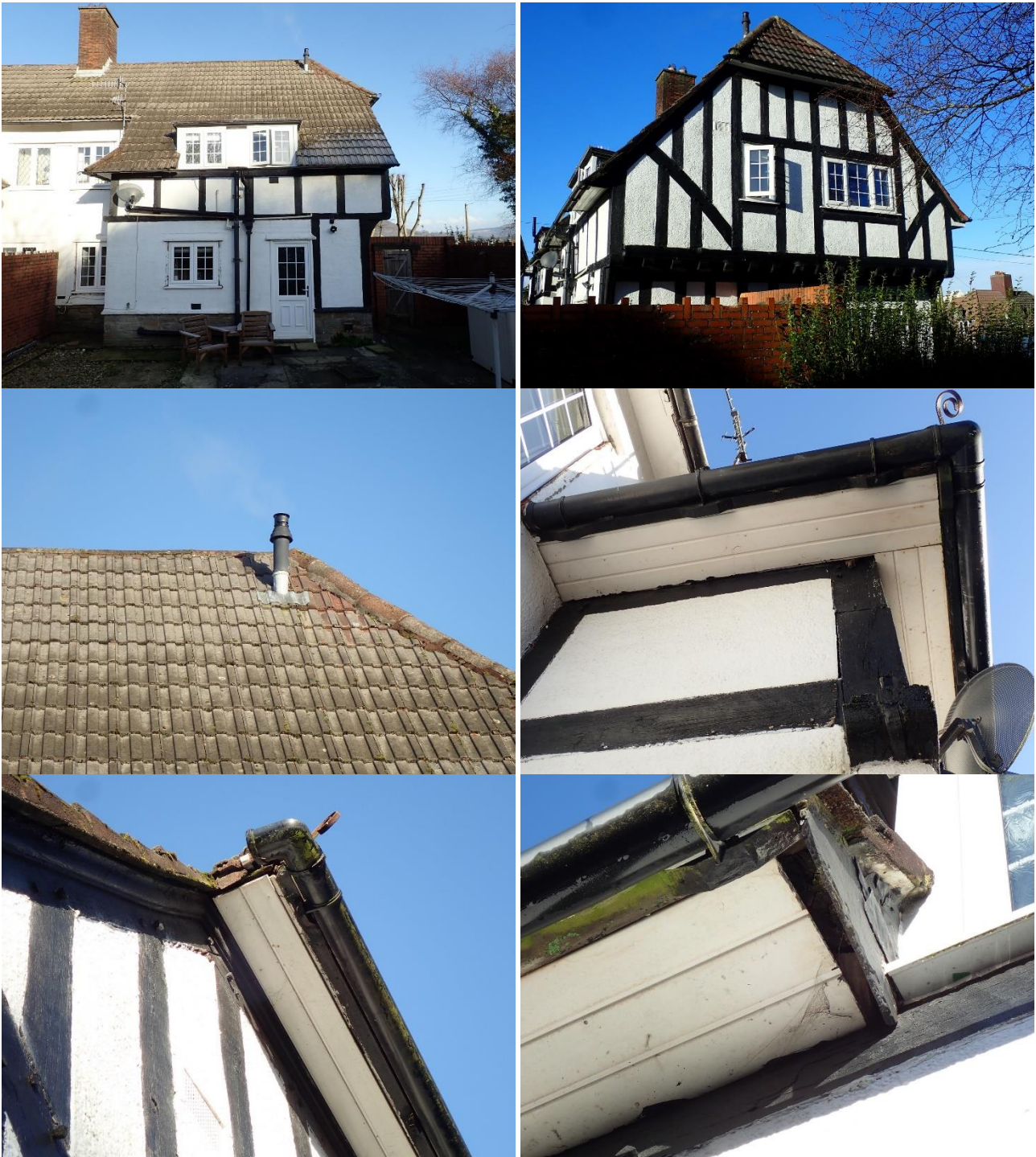
External photographs (Clockwise from top left): South elevation with dormer windows; eastern elevation with timber and beam structure and hipped roof; minor squeeze gaps behind soffit box; potential access into soffit box adjacent to dormer window; base of hipped roof on eastern elevation; well-sealed flue adjacent to well-mortared hip tiles.
