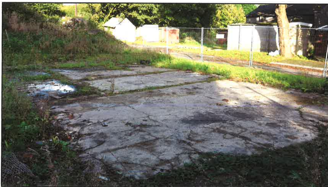
Plate 3: Centre of the Site – former building floor slab. Lane in background.
