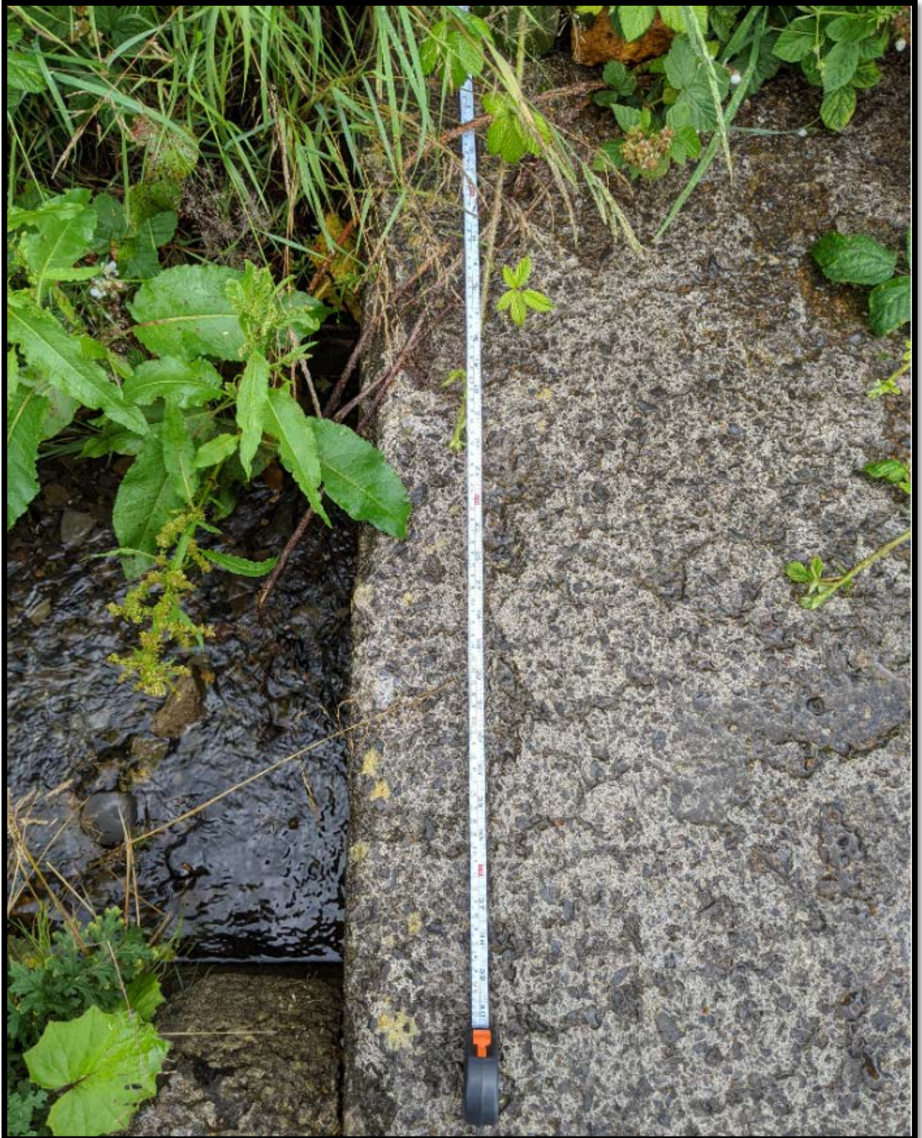
Photo 3: Shows the taped measured width of the existing Culvert
