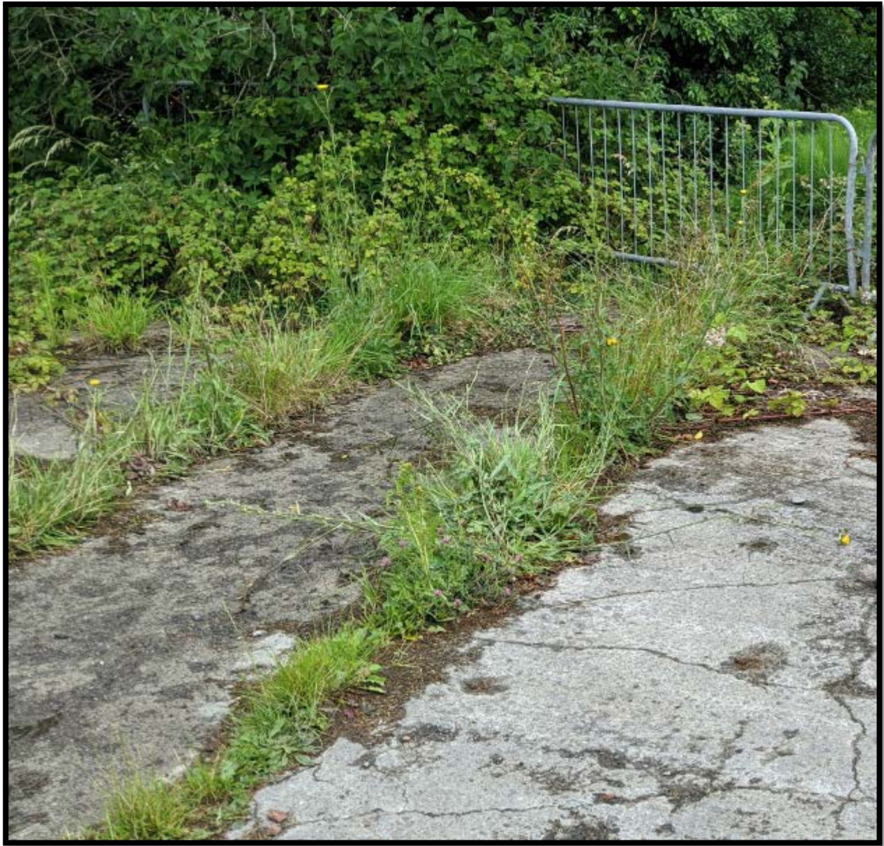
Photo 4: Shows the extent of the existing culvert cover slab in the road crossing.
