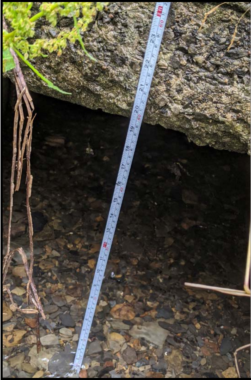
Photo 1: Shows taped measured dept of existing culvert from soffit of cover slab.
