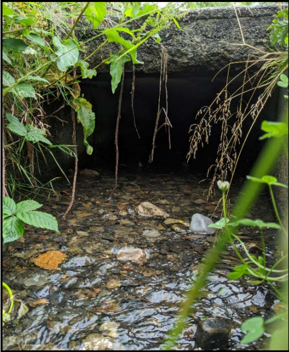
Photo 5: Shows the outfall of the existing culvert.
