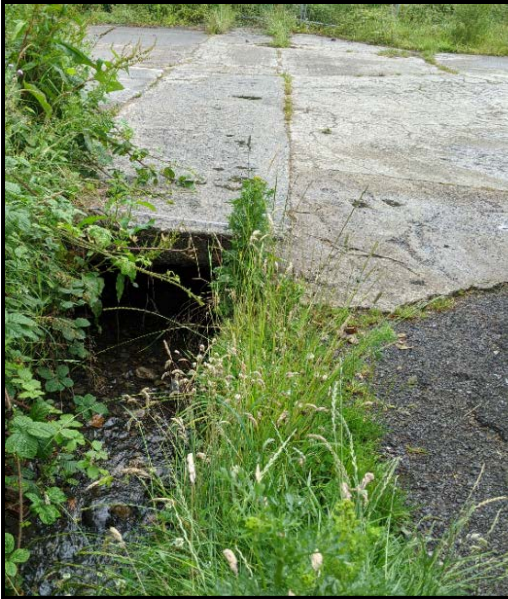
Photo 6: Shows the outfall of the existing culvert and the road crossing.
