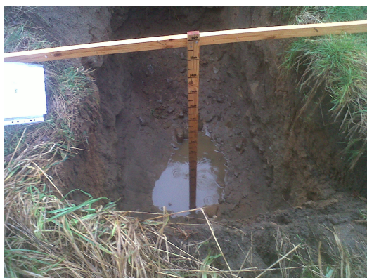
Photograph shows Trial Pit 2 after 120mins with only a small amount of water remaining < 25mm.
