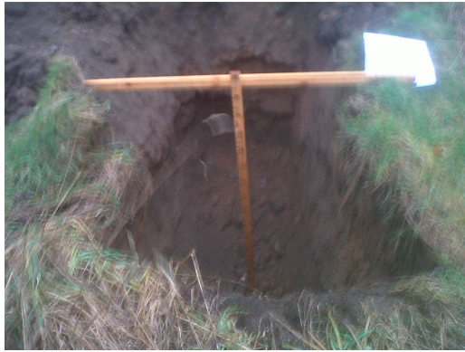
Photograph shows excavated Trial Pit 2 with 1600mm long timber measuring tool resting on base and top edges.
