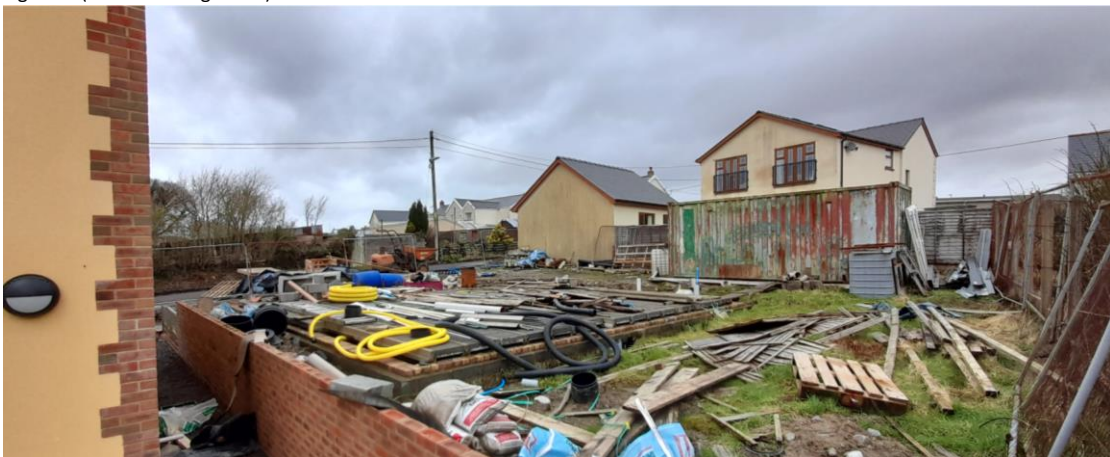
Figure xii (Slab – Looking north)
