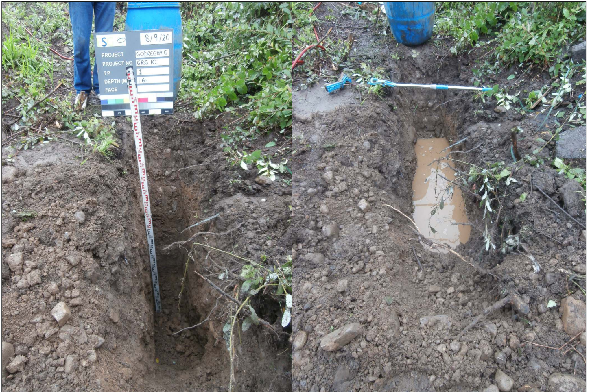
FIGURE 1 SOAKAWAY PIT ON EXCAVATION AND DURING TEST
