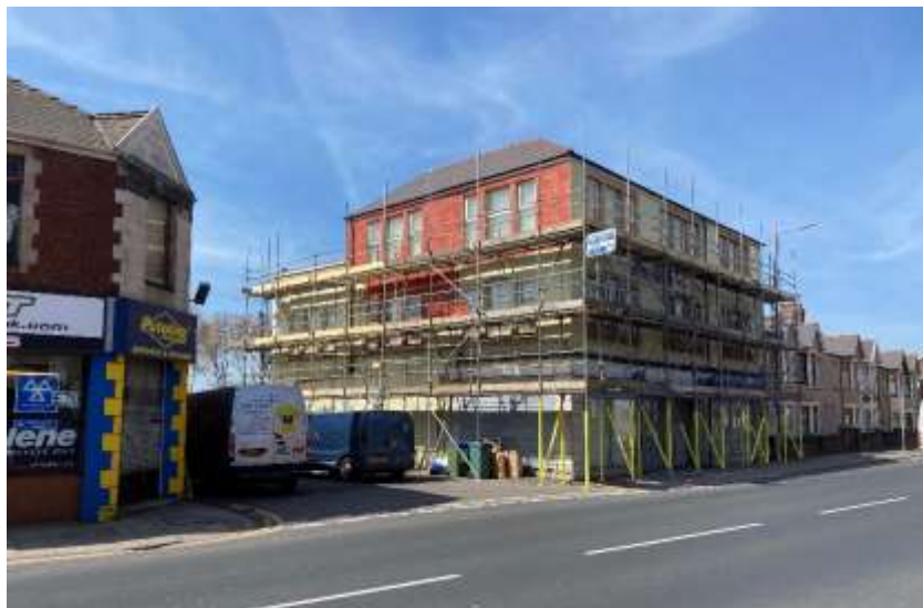
Photo 2 – view looking west towards application building
