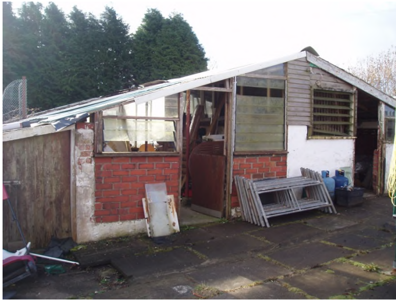
Showing buildings 1b
