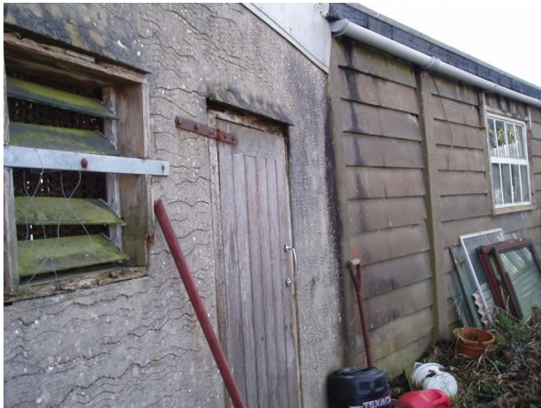
The tool shed and concrete buildings (nos 2 and 3)
