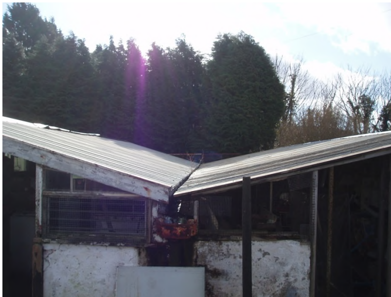
Roof valley between building 1a and 1b
