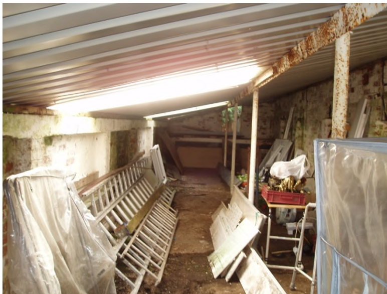
Building 1a interior
