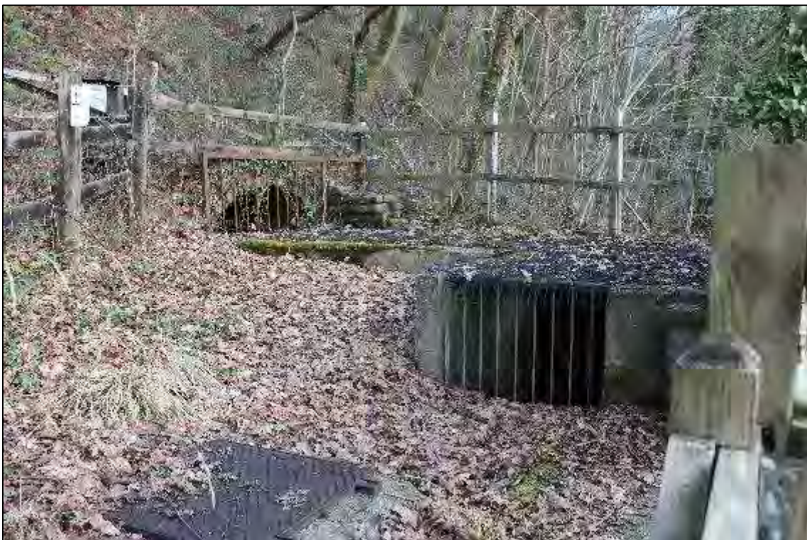
Plate 6: Probable former coal level (Asset 4), Area A, facing north
