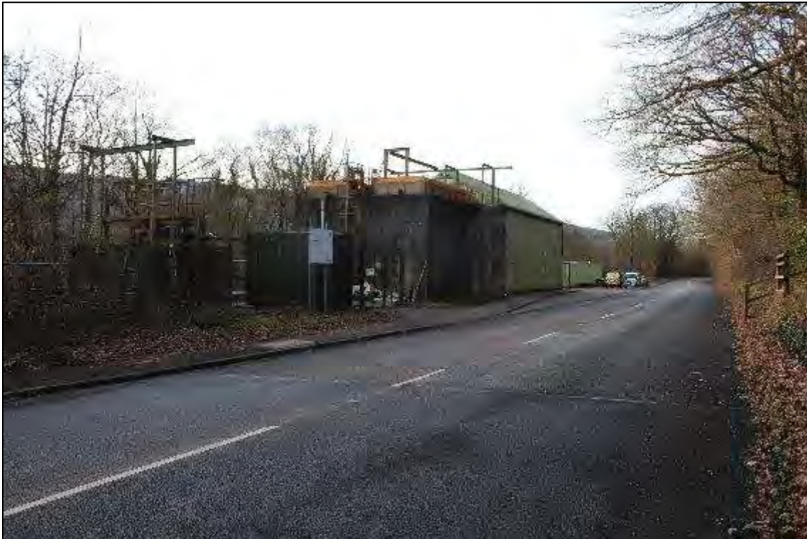
Plate 5: Existing Ynysarwed Plant structures, Area A, facing south
