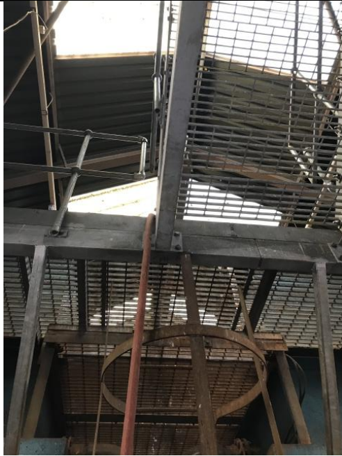
Photograph 34: The interior of Building 3 showing the lack of insulation on the roof.
