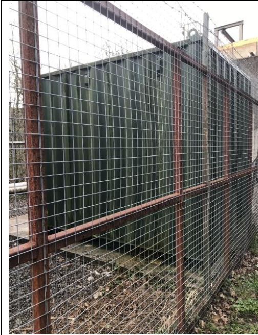
Photograph 38: The north east face of Building 5.
