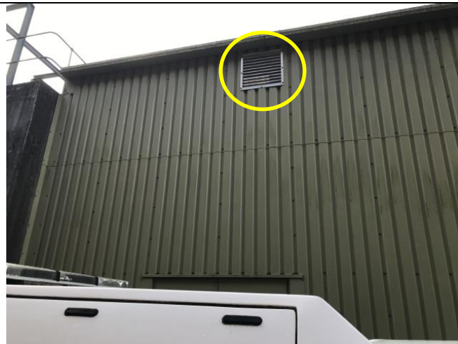
Photograph 32: The location of the vent on the north west face of Building 3.
