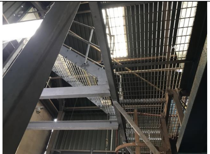
Photograph 33: The interior of Building 3, which is well lit and surrounded only by corrugated metal walls.
