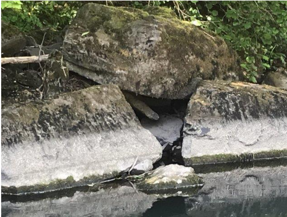
Photograph 1. Otter holt recorded on bank of River Neath
