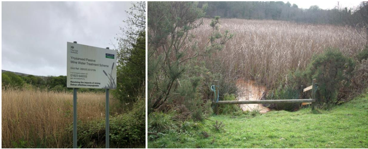
Photograph 7 – The passive reed beds
