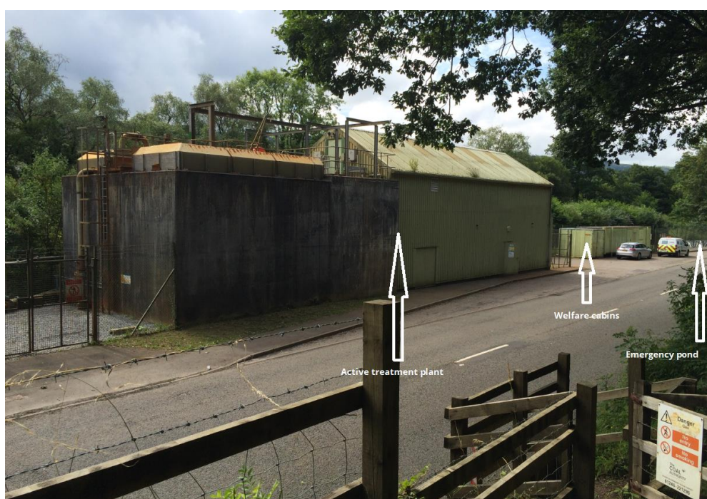
Photograph 6 – The existing active treatment plant
