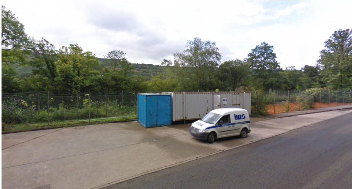
Photograph 9 – Existing office/welfare facility
