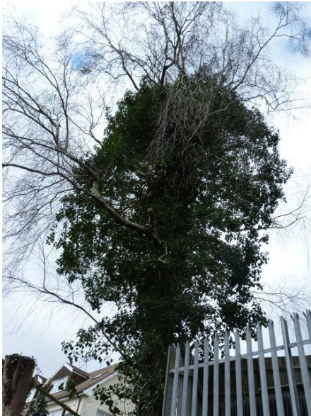
Figure 17: Birch tree growing adjacent to electricity sub-station.
