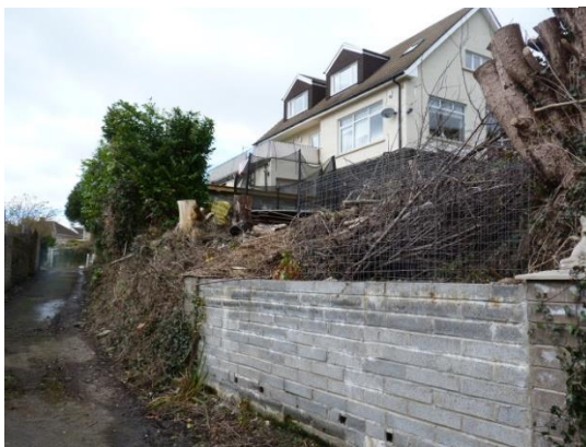
Figure 25: Landscape to the south of the project site (on the right hand side)
