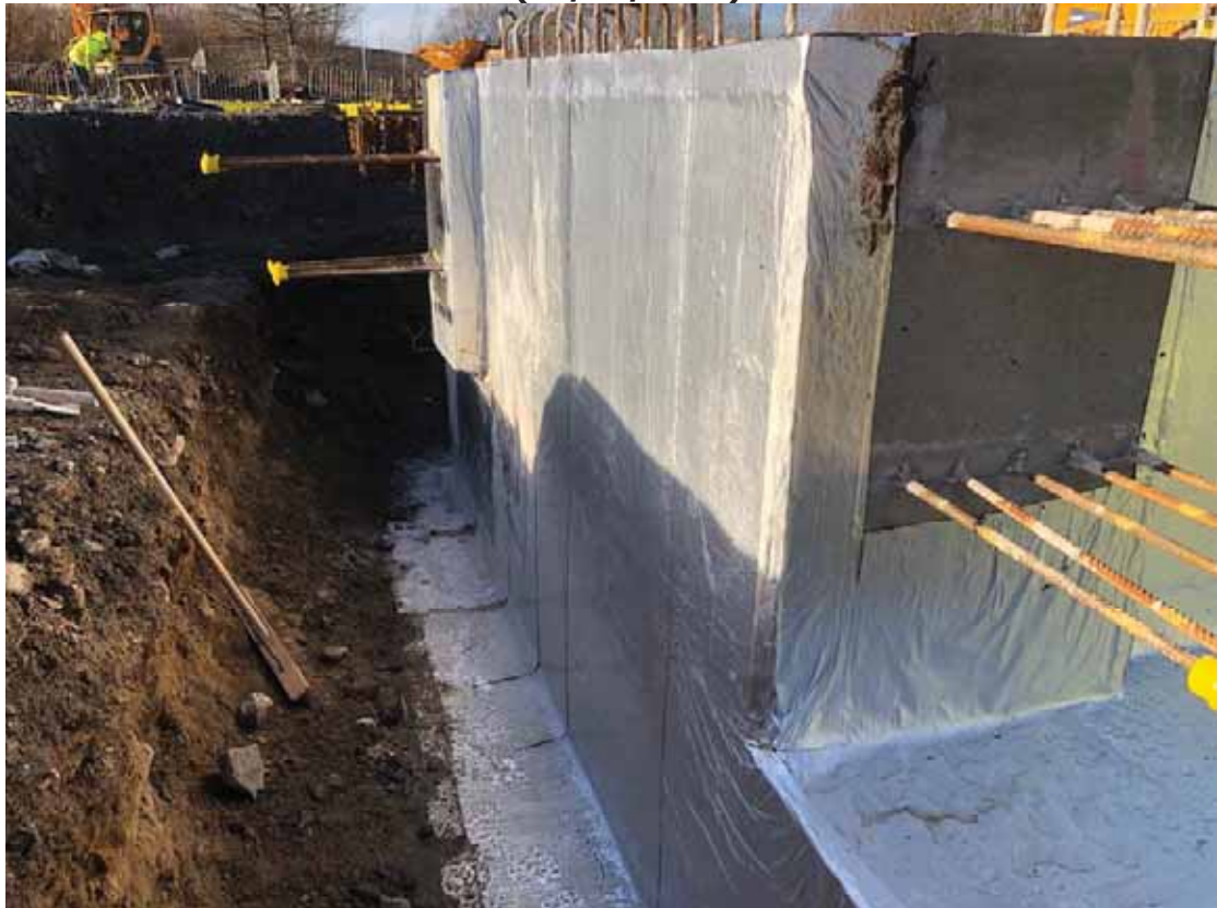
Plate 2 Lift Shaft – Visit 1 (15/12/2020)
