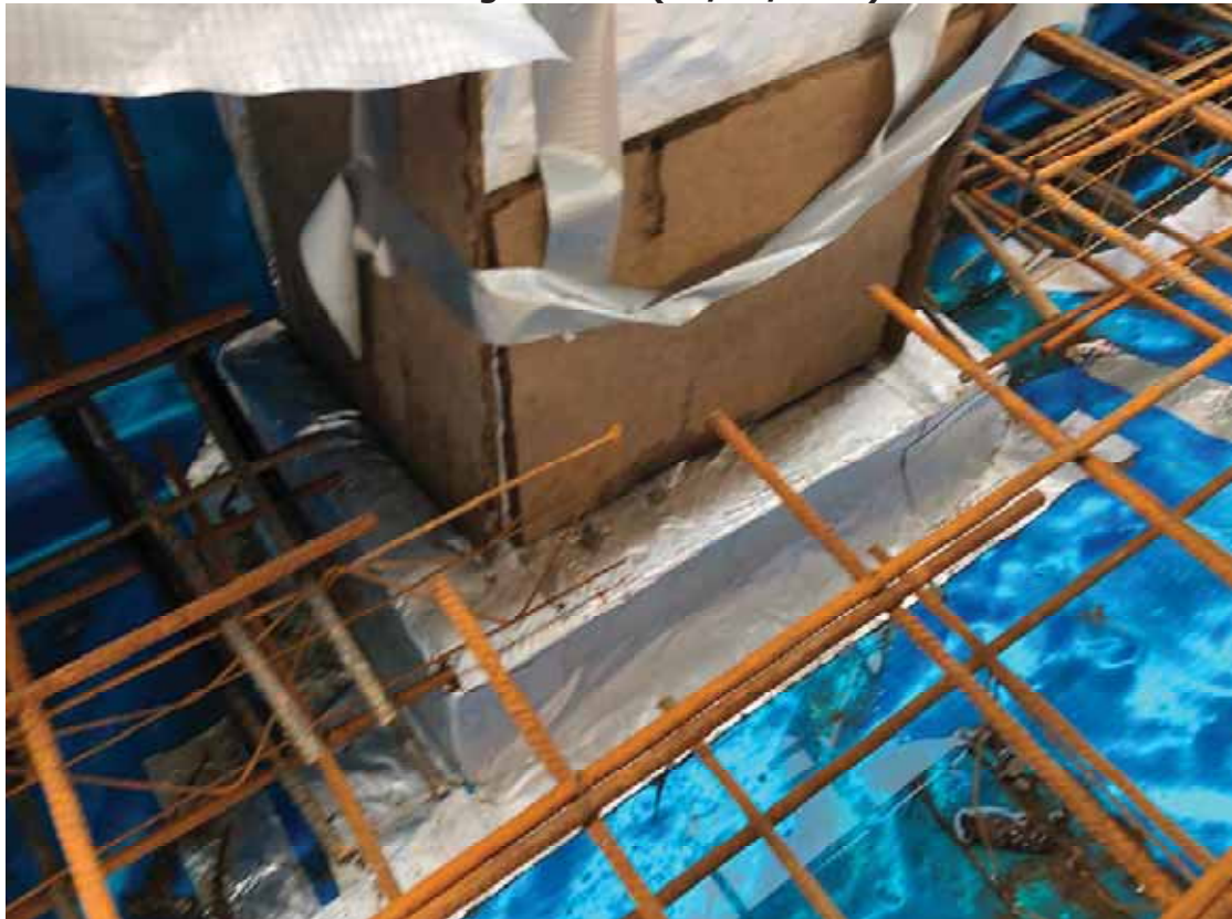
Plate 12 Column Detailing – Visit 3 (08/04/2021)
