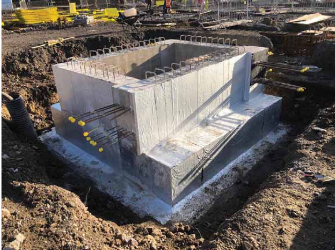
Plate 1 Lift Shaft - Visit 1 (15/12/2020)
