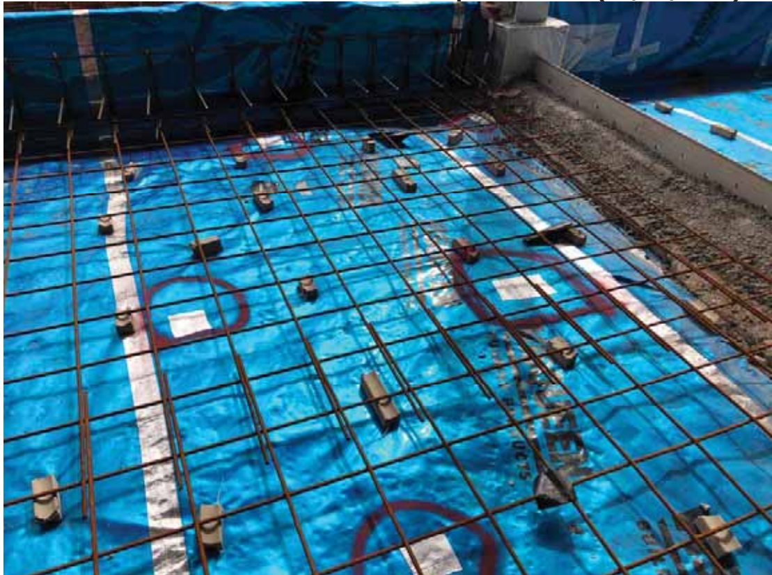
Plate 10 Membrane Installation with Repairs– Visit 2 (01/04/2021)
