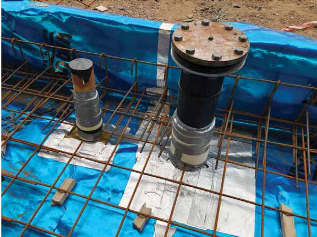
Plate 7 Sealed Penetrations – Visit 2 (01/04/2021)
