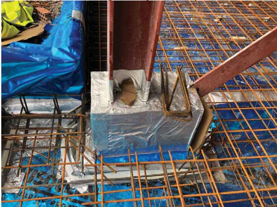
Plate 8 Column Detailing - Visit 2 (01/04/2021)
