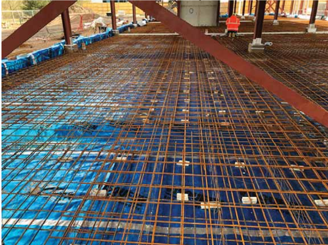
Plate 11 Membrane Installation – Visit 3 (08/04/2021)
