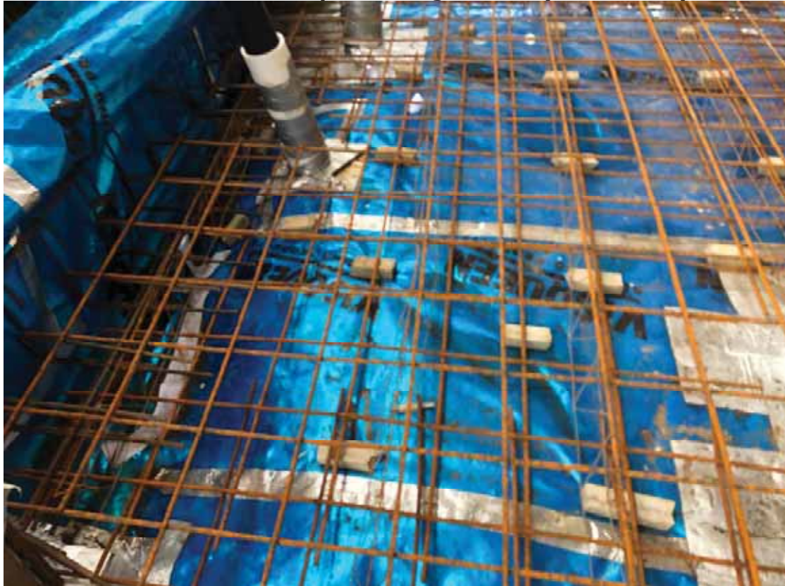
Plate 13 Membrane and Pipe Detailing – Visit 3 (08/04/2021)
