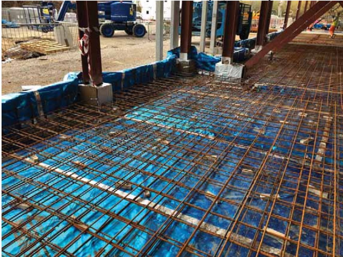
Plate 6 Membrane Installation – Visit 2 (01/04/2021)
