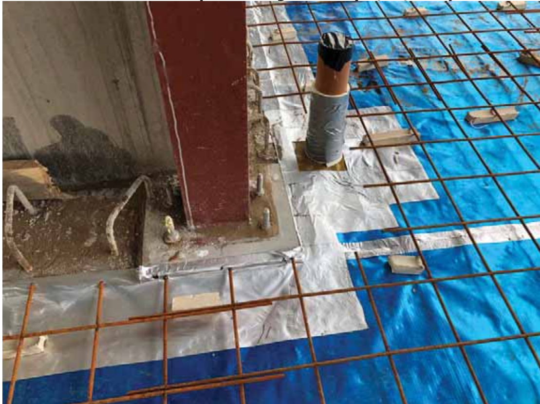
Plate 4 Column and Pipe Detailing – Visit 2 (01/04/2021)
