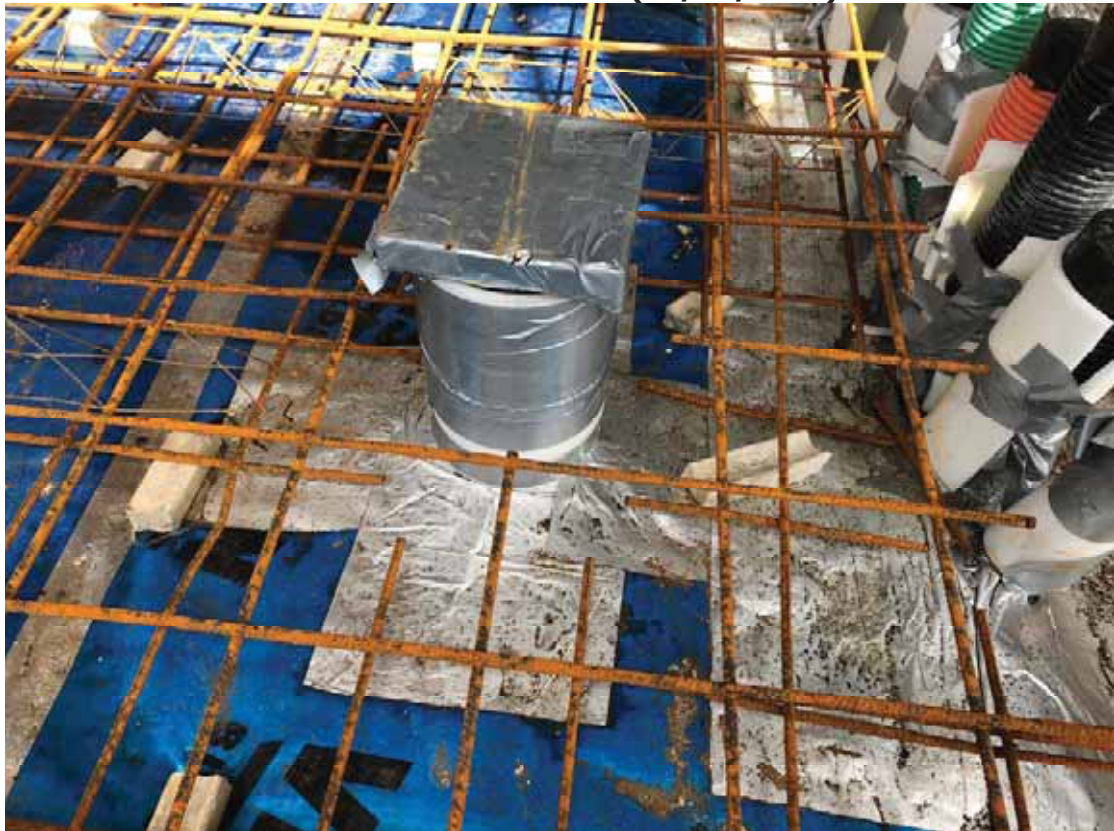
Plate 14 Sealed Penetrations – Visit 3 (08/04/2021)
