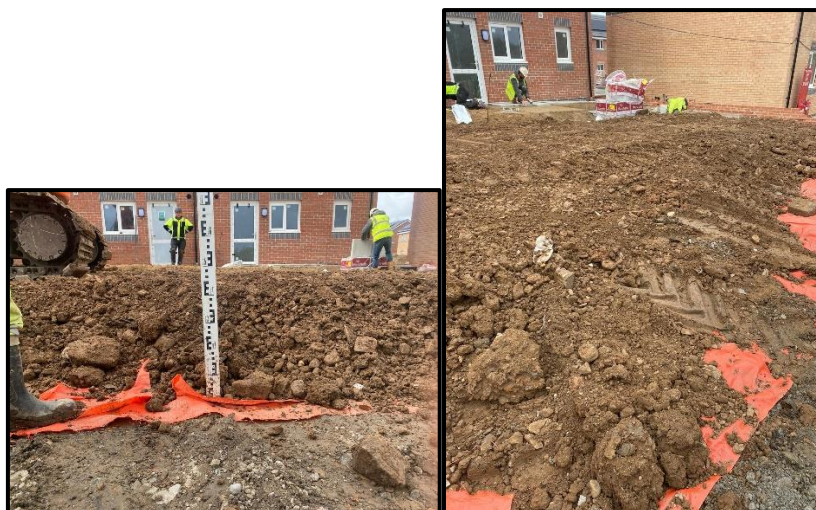
Plates 02 & 03. Placement of Subsoil prior to compaction and placement of 'Topsoil' layer.
