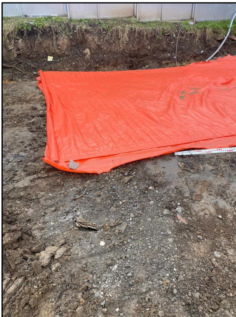
Plate 01. No-Dig Barrier being set out at -600mm
