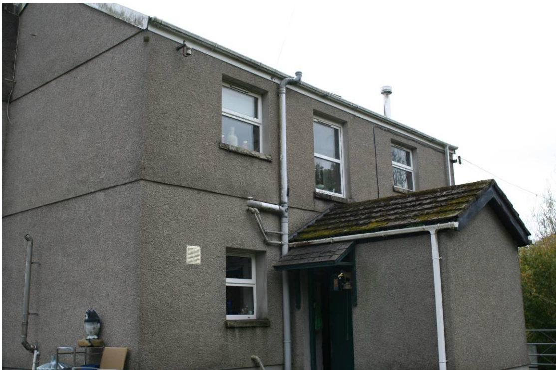
SW Elevation of building
