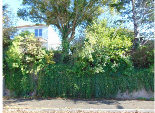
continuation of retaining wall frontage to east of no. 14
