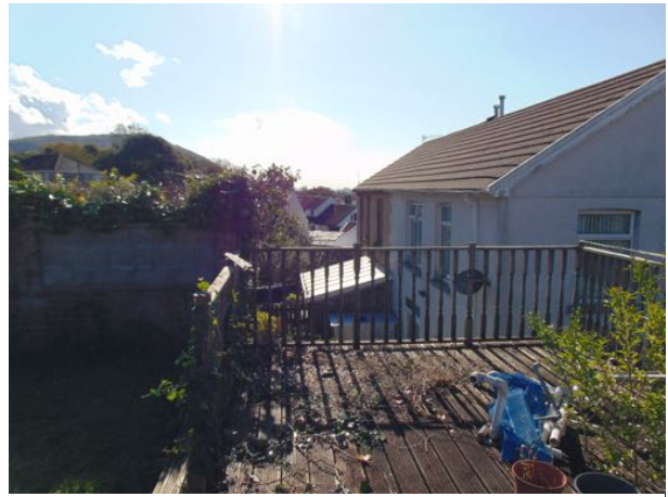
adjacent view – to no.8 – looking east
