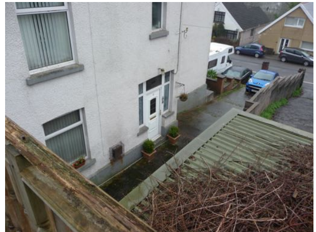
view 2 from deck to entrance to no. 8
