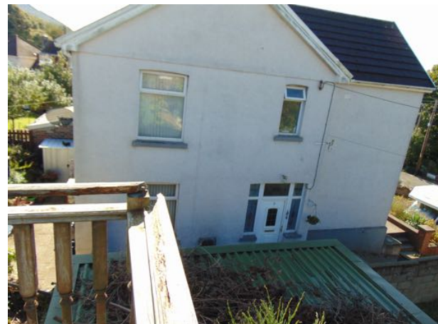
adjacent view from scaffolded deck towards no. 8
