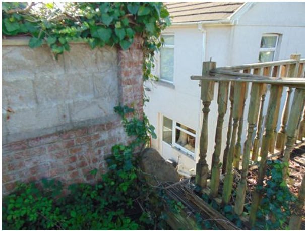
Boundary junction: nos. 8 & 14 at garage block & deck over
