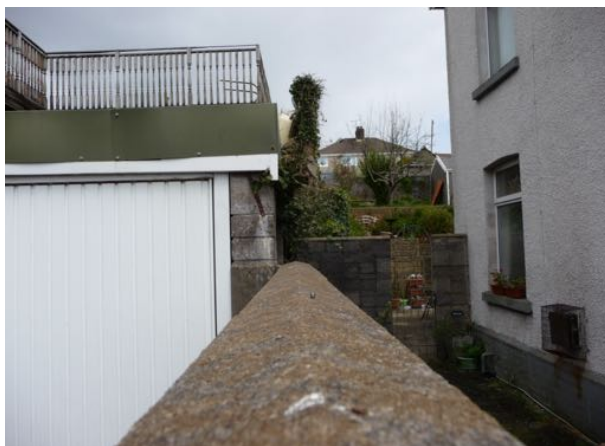
view at retaining wall coping level along boundary against no. 8 entrance
