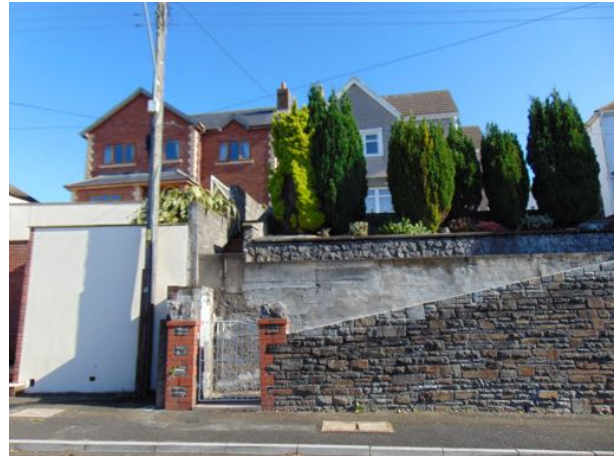
retaining wall frontage of existing houses 16/18 Old Rd
