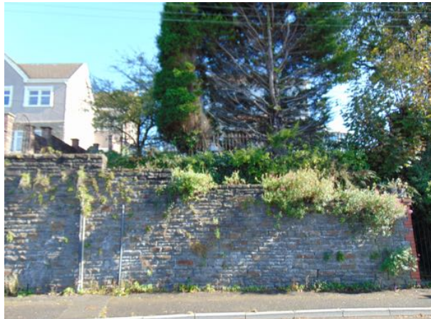
continuation of frontage retaining wall to no. 14
