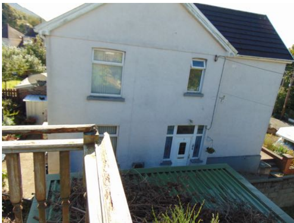
view from deck down to no. 8 entrance area
