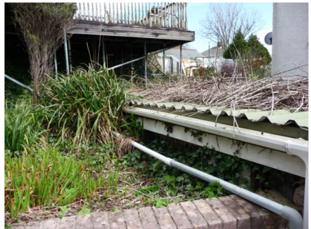
view over garage roof to rear corner of no. 8
