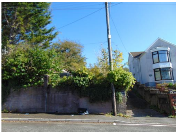
last section of frontage retaining wall before access drive
