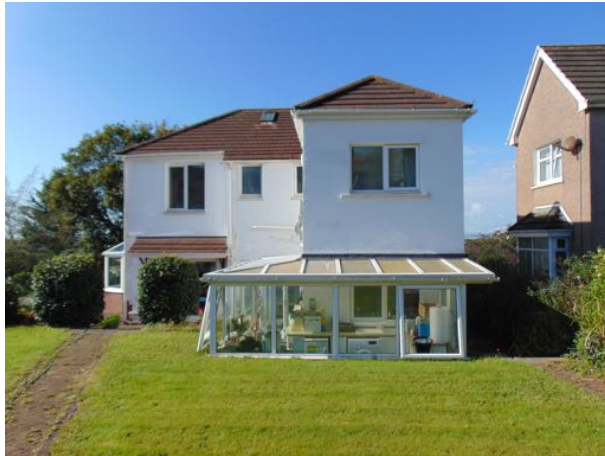
north elevation of existing house from annexe
