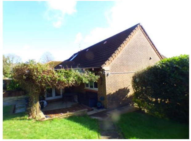
view to E close up of side of existing house
