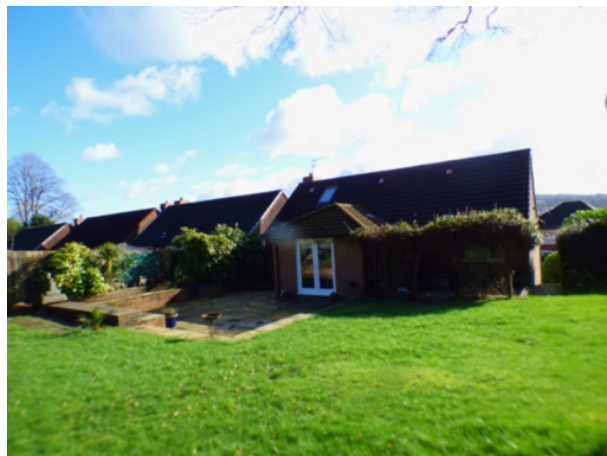
rear north-facing elevation of existing house
