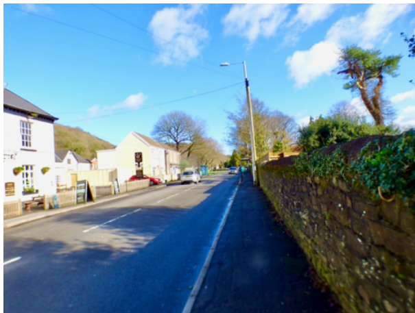
Main Rd frontage wall (to be lowered) from NW site corner
