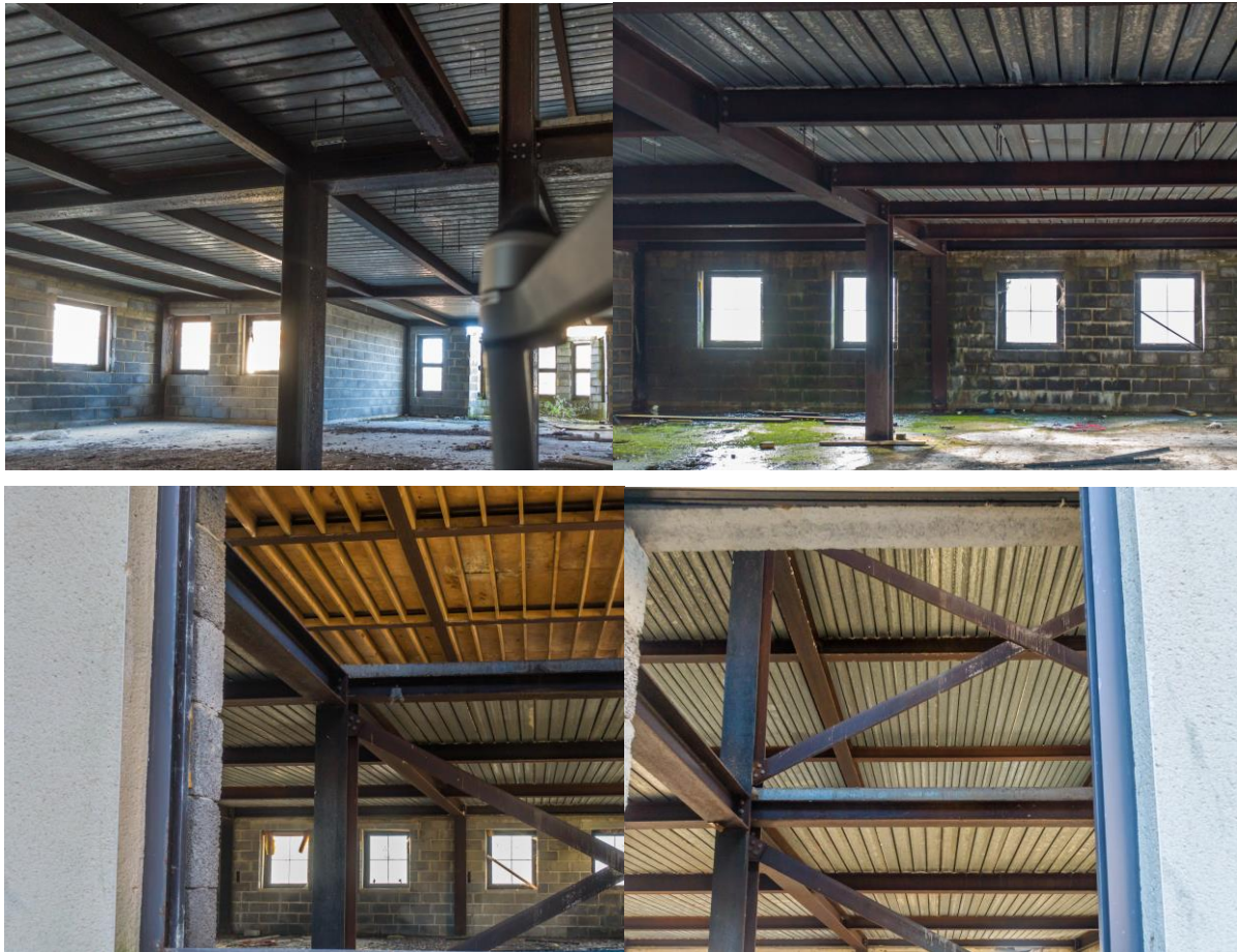
Images of the upper floors with post and beam ceilings. You can also see the timber floor of the roof space.
