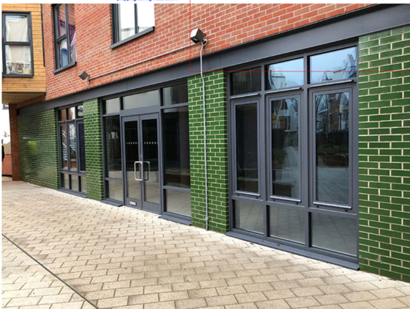
NEW DARK GREY ALUMINIUM SHOPFRONT WITH GLOSS GREEN BRICK SLIPS
