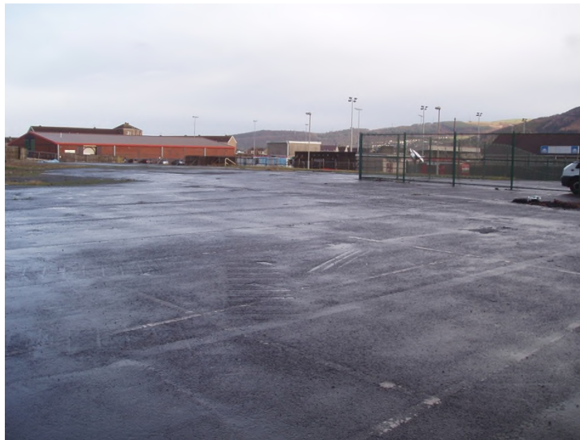
Looking north west across Lido Site
