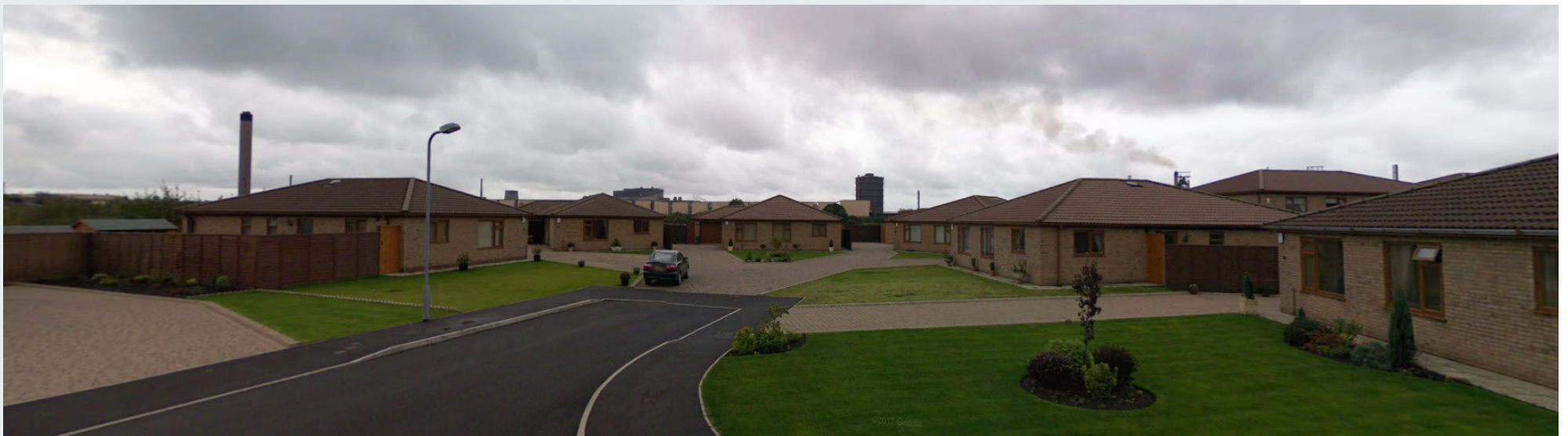
Figure 18 - Stallcourt Close (Google Maps)
