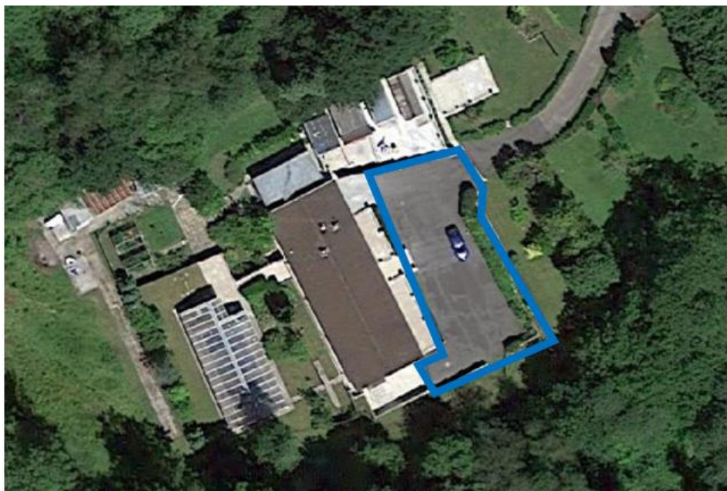
Blue line showing the approximate area of parking on the site
