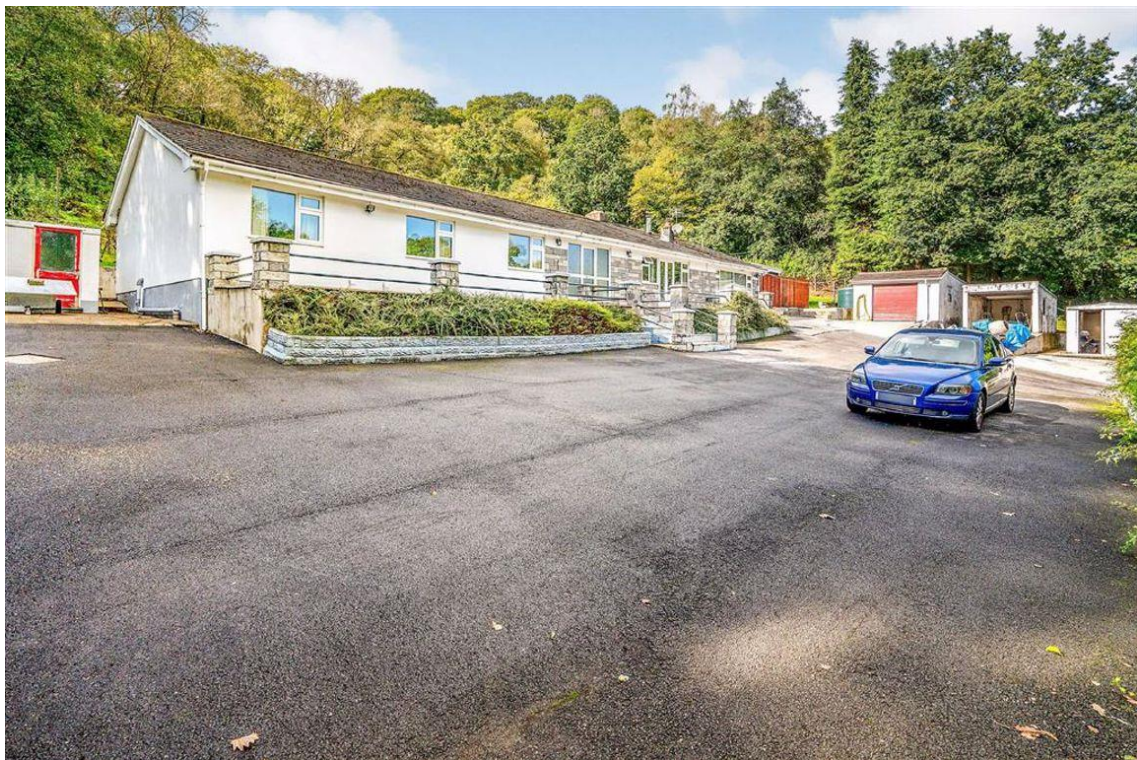
View of the dwelling and driveway
