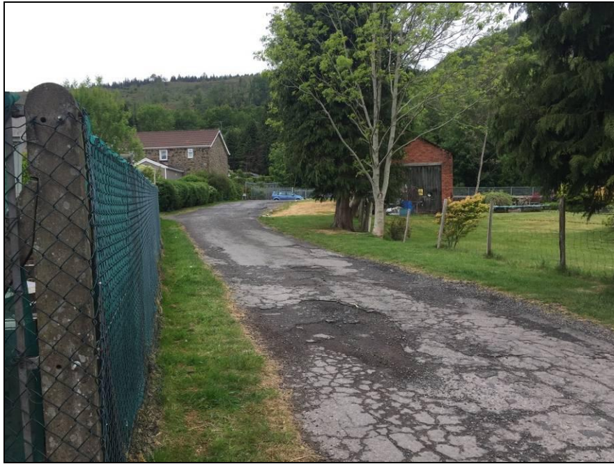
Figure 9. Tarmac access track with grass verges
