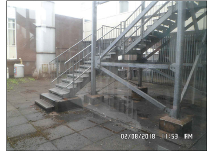
EXTERNAL FIRE ESCAPE
