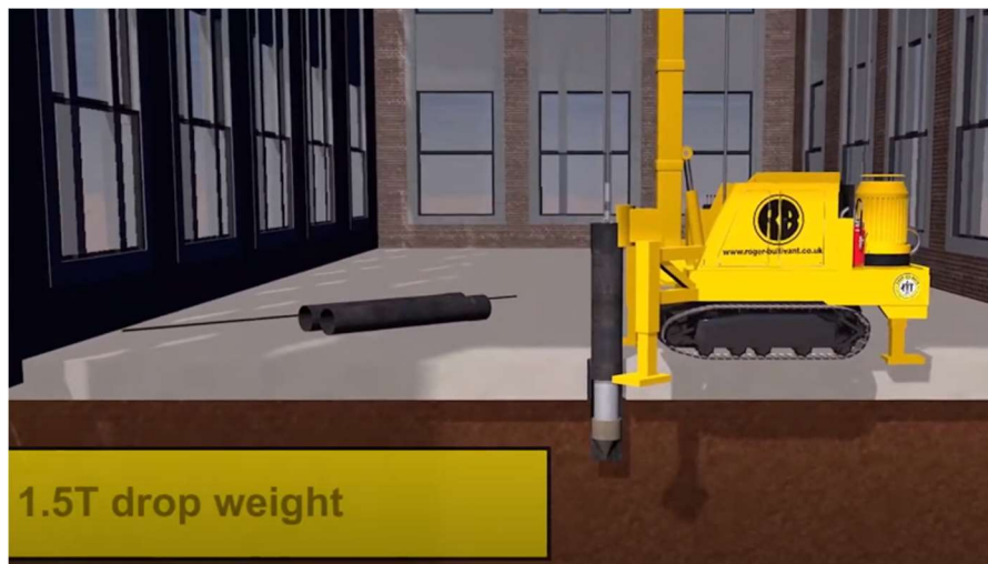
Figure 1 : Driven pile installation process
