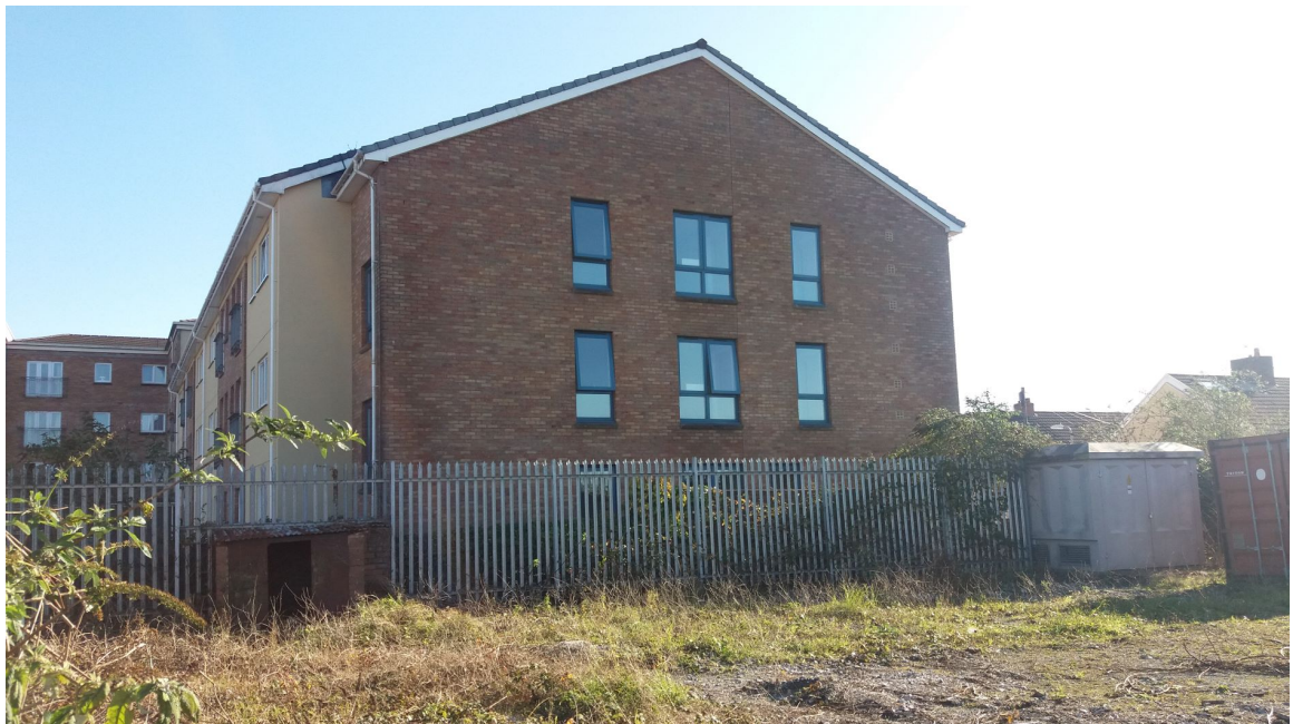
P4. VIEW EAST ON REAR SITE SECURITY FENCE
