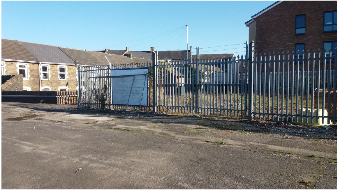
P3. VIEW EAST ON ACCESS GATES TO SITE AND SECURITY FENCE
