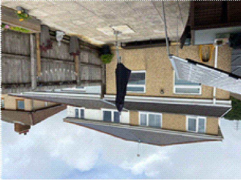
Existing image of rear elevation showing neighboring property.
