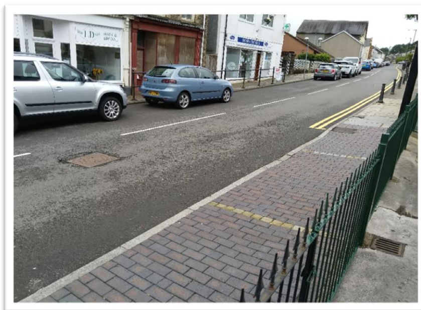
LEFT: Existing long length of dropped curb footway crossing and contrasting demarcation paving line illustrates the past use of the forecourt area for retail parking in past times when the area was very much busier and demand for parking at a premium. Decorative metal fencing added in recent years to prevent disturbance from unauthorised parking.
