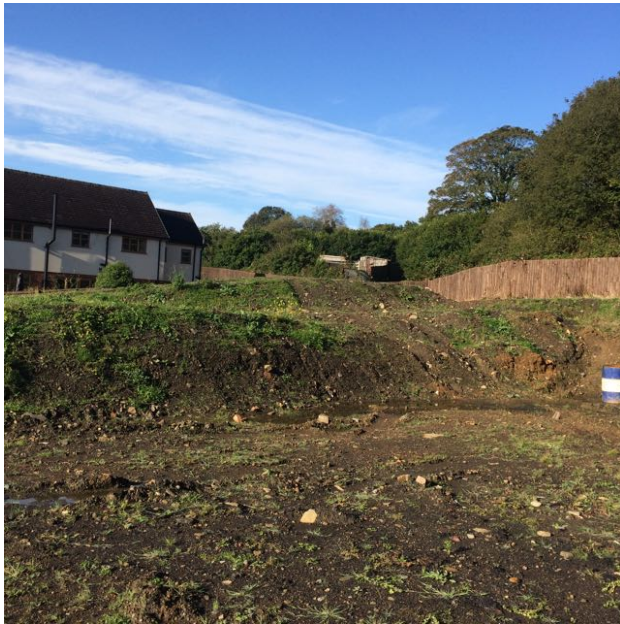
Figure 3. Bunds at western end of site.
