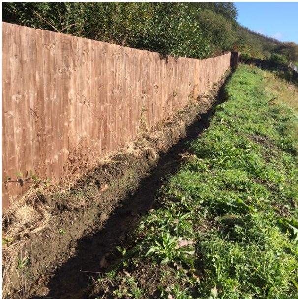
Figure 5. Drainage ditch on northern boundary.
