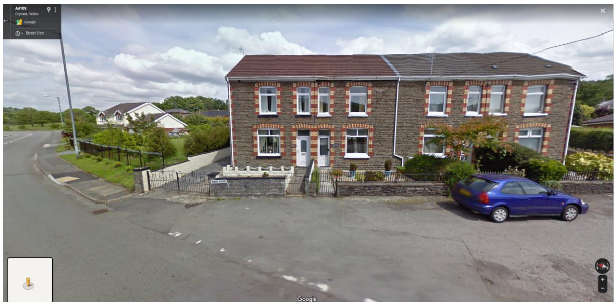
Figure 3 - Photographs showing terraced houses adjacent to site.
