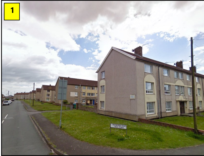
View of flats looking along Moorland Road
