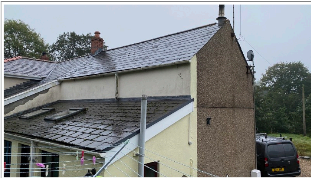
Photo 2: North-east and north-west facing elevations of the main dwelling with lean to
