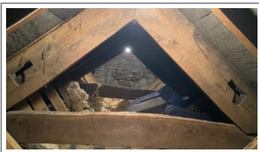
Photo 5: Shallow roof void of main dwelling
