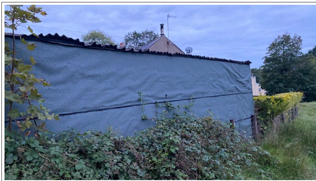
Photo 7: West facing elevation of garage
