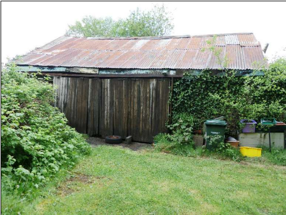
Photo 24: Southern stone barn with corrugated pitched roof.
