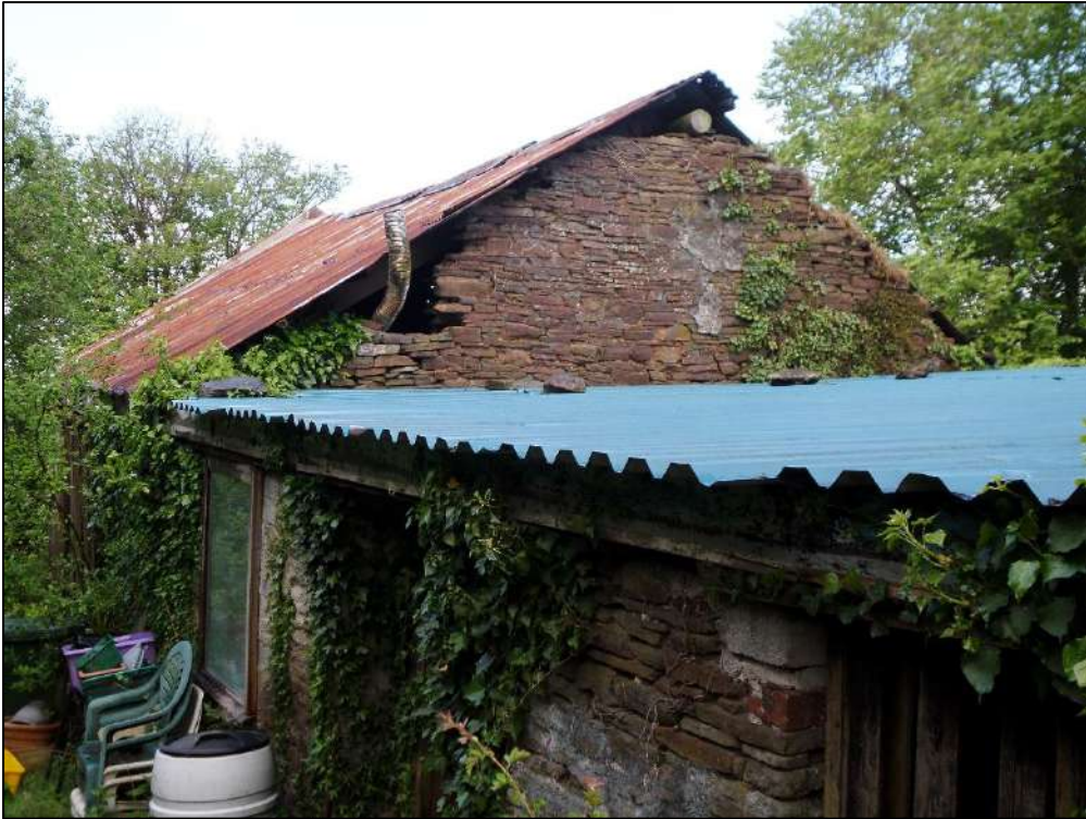
Photo 25: Northern stone barn with a mono pitched roof.
