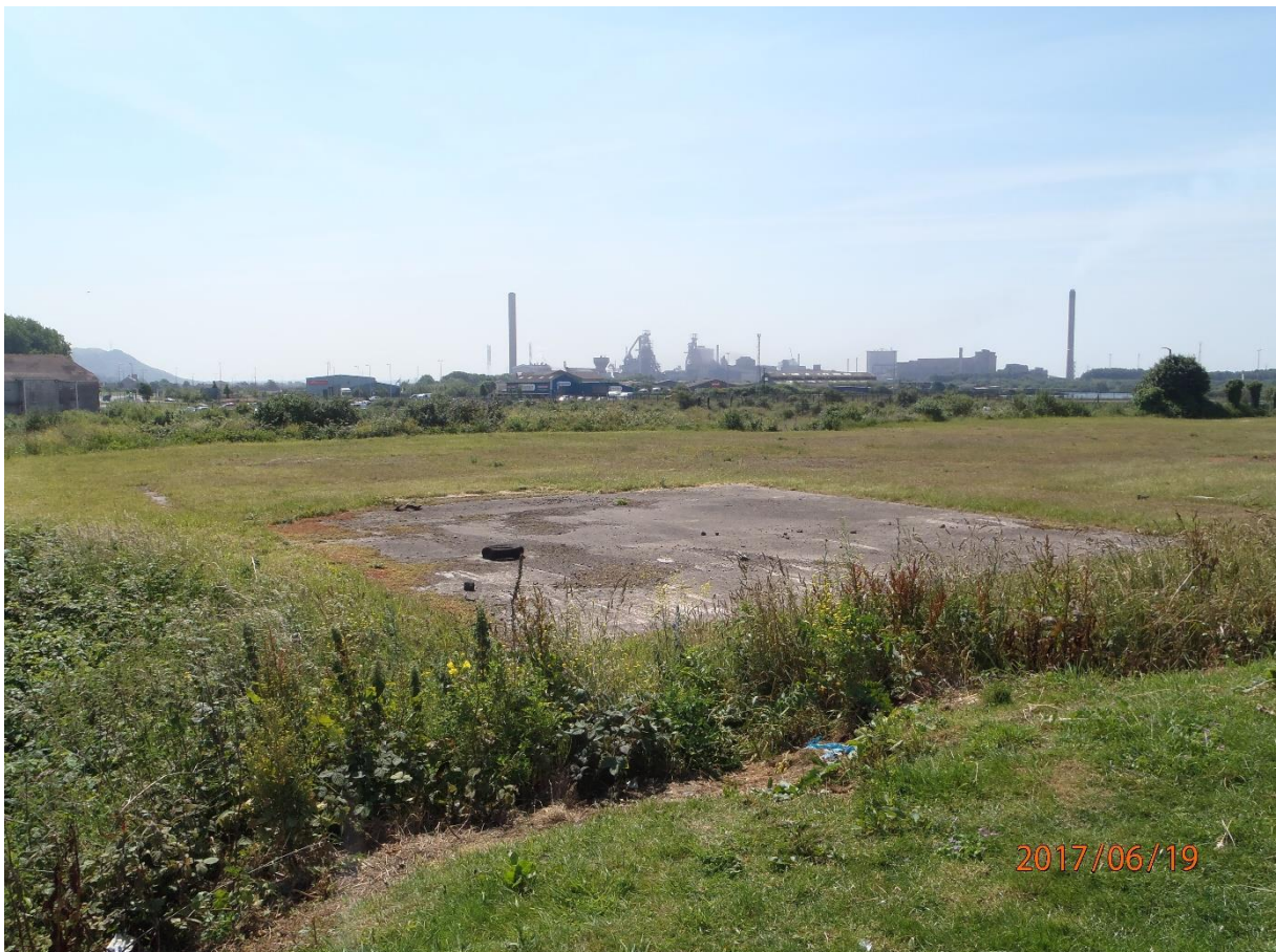
Plate 12: View looking south east across west of site from earth bund showing raised area and concrete hardstanding
