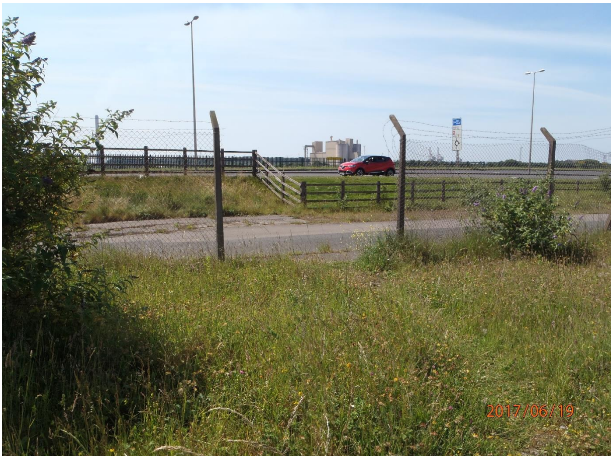
Plate 24: View of southern boundary fencing and missing section on "Dock Road" (approximately 3.5m between posts for access)
